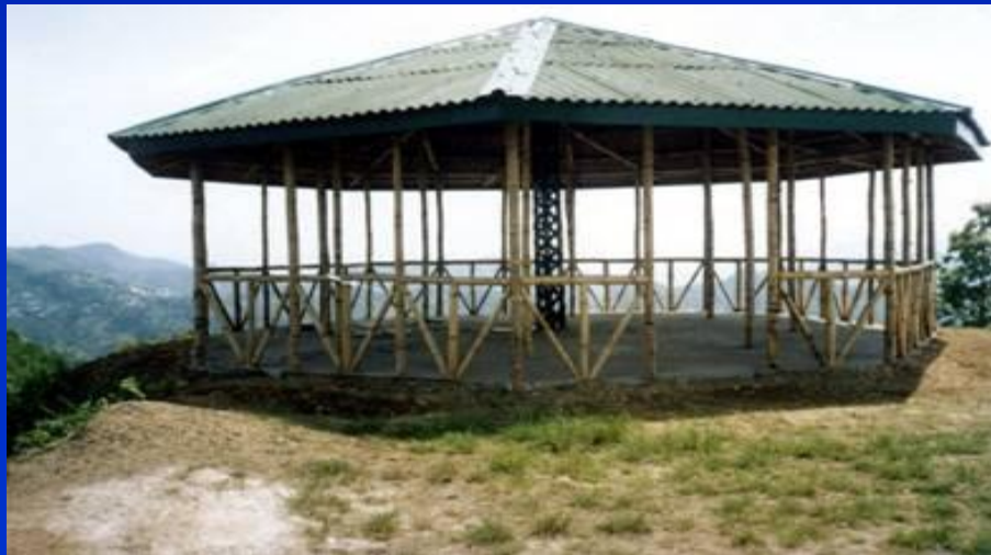
Picnic Hut at Tiangnuam, Aizawl - COMPLETED
