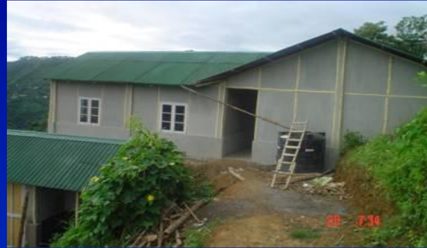
School Building at Aizawl. - COMPLETED
