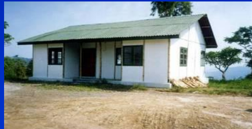
Type II house at Luangmual, Aizawl - COMPLETED
