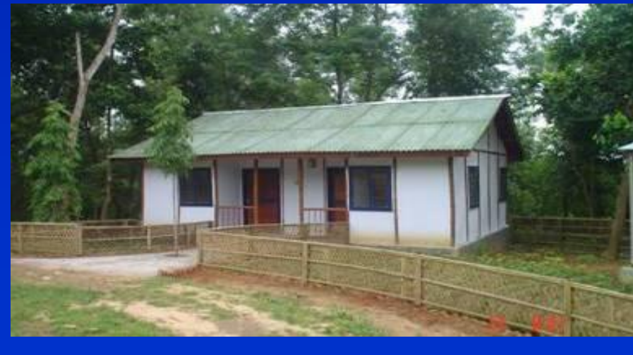
Type II house at Circuit House Udaipur - COMPLETED
