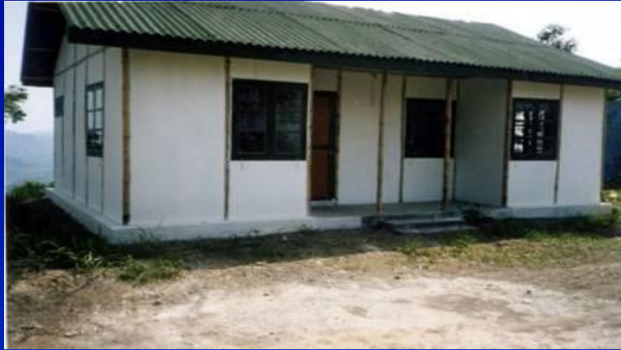
Type II house at Lunglei. - COMPLETED
