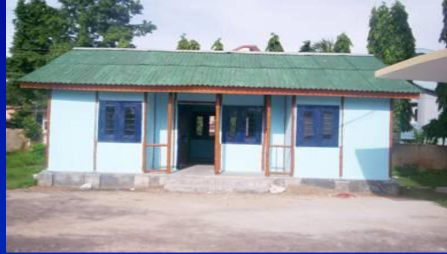
Type II house at Circuit House Agartala - COMPLETED
