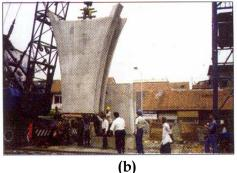
**Figure 11:** Massive Pre-cast Piers used for flyovers without disruption of underlying services and utilities: (a) JJ Hospital Flyover on Precast Piers in Delhi, and (b) Transportation of Precast Piers from site of construction to erection site (Bhattacharya, 2002)
