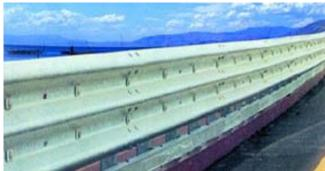
Figure 10: Steel Guardrail Systems (Source: www.kirby-india.com, 2004)
