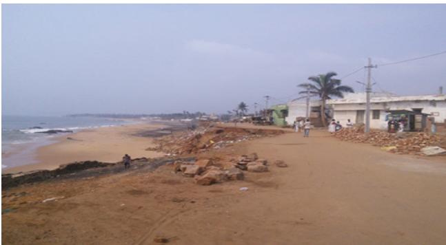
Image 3: Damaged Road during Cyclone Hud-Hud near Bhimunipatnam
