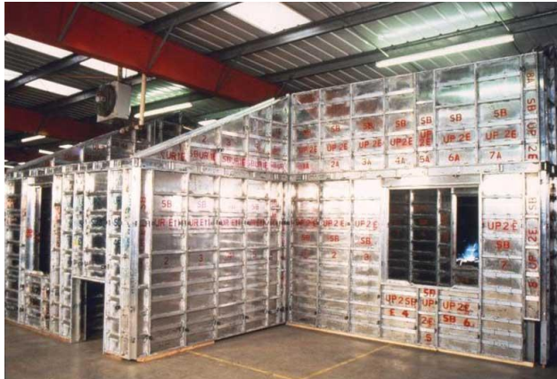
Fig 11: View of MIVAN formwork [37]
