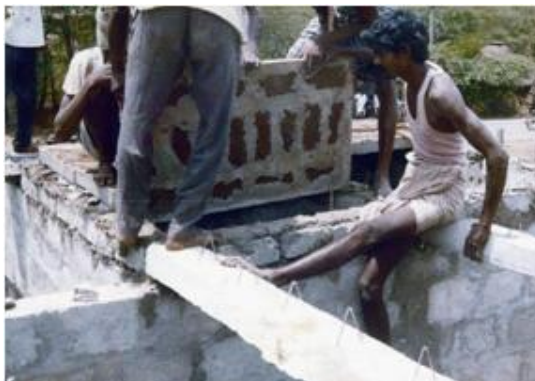
Fig3: Laying of brick panel [15]
