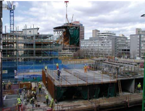
Fig 12: Tunnel formwork [41]
