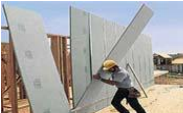
Fig13: View of gypsum area separation wall [67]
