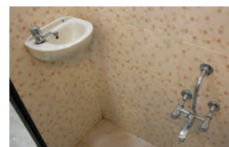
ATTACHED TILED BATHROOM & TOILET
