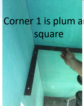
Wall 2 Panel 1 sits on base plate up against the post 1 creating corner 1
