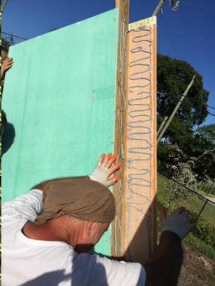
Panel 1 sits on base plate up against the post 1
