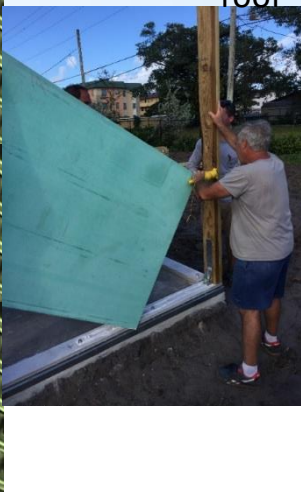
Wall 1 Panel 1 sits on base plate up against the post 1
