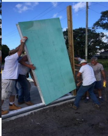
Wall 1 Panel 1 sits on base plate up against the post 1
