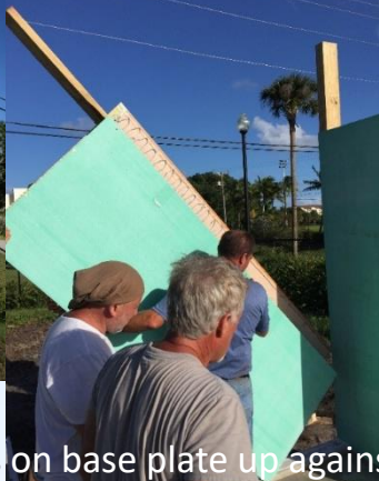
Panel 1 sits on base plate up against the post 1
