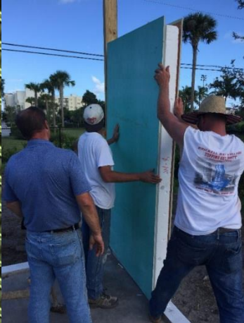
Panel 1 sits on base plate up against the post 1
