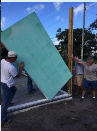
Wall 1 Panel 1 sits on base plate up against the post 1
