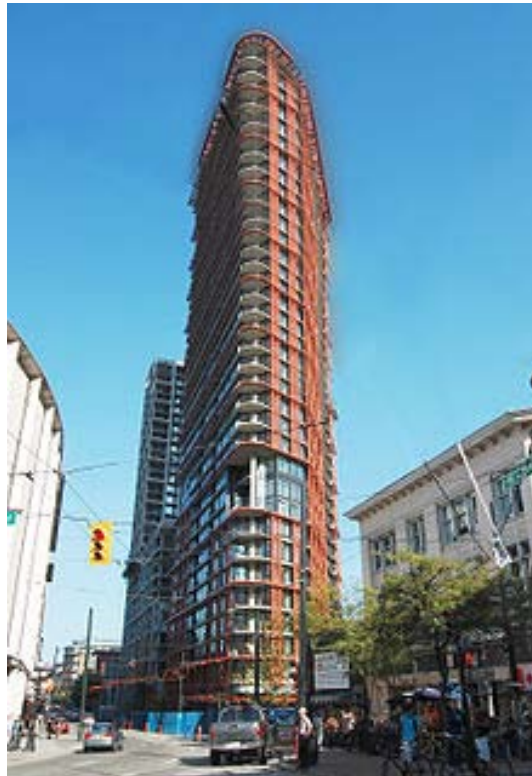
Figure 3.21: Woodward's redevelopment project in Vancouver, BC by Henriquez Partners Architects (Source: http://henriquezpartners.com , nd).
