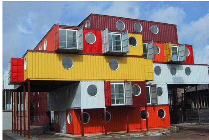
Figure 4.62: Container housing can be stacked up to 5 stories without structural reinforcement; Container City in London (Source: http://www.choices.co.uk , 2012).
