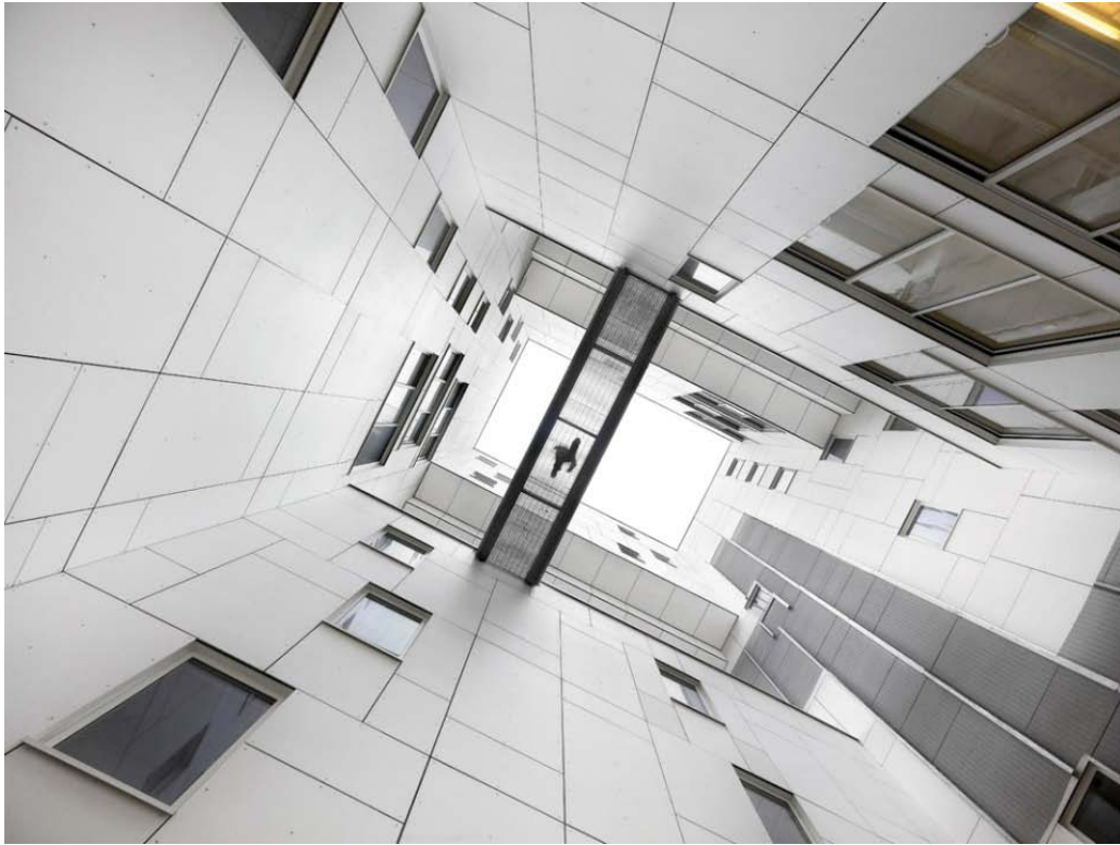
Figure 3.57: The void core opening from the second floor to the building's full height brings natural ventilation and light into all units (Source: ArchDaily, 2010).
