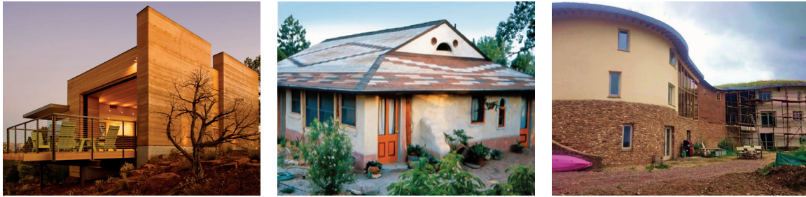
FIGURE 1. Rammed earth house in Arizona (The Construction Zone, 2008) (left), earthbag cottage in Utah (Kennedy, 2012) (middle), and Cob house in UK (Maccabe, 2010) (right).
