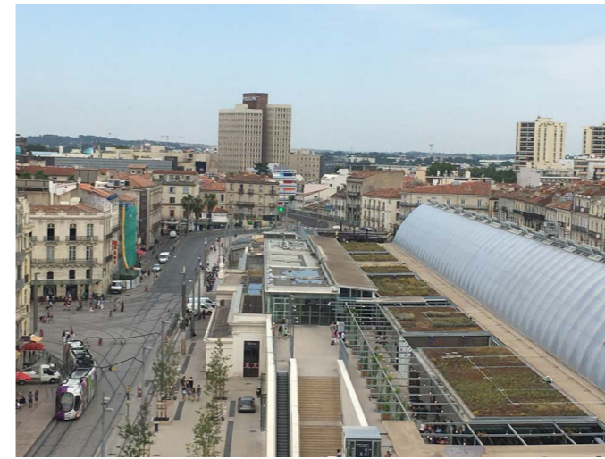
THE STATION HAS BEEN TRANSFORMED
