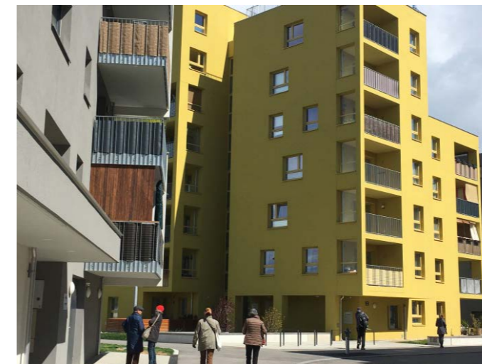
MEDIUM RISE MODERN APARTMENTS
