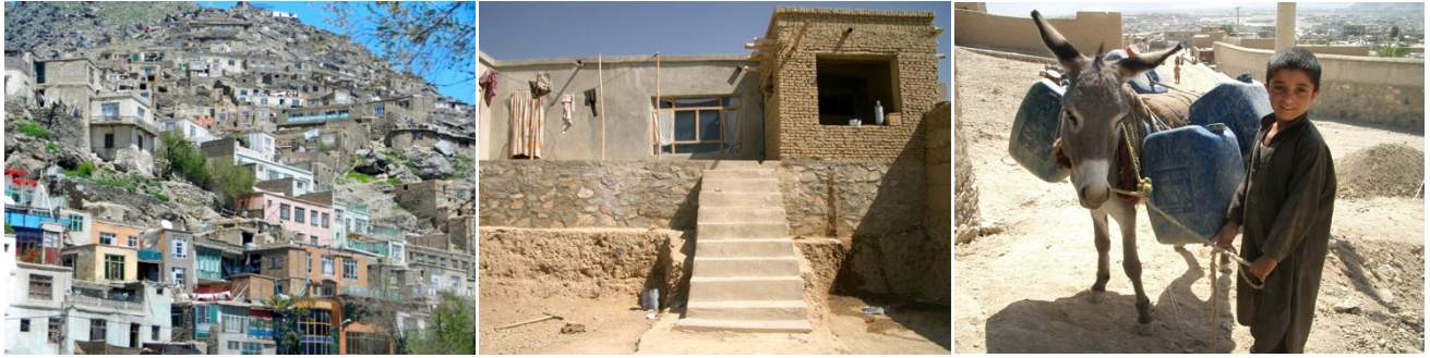
Left: Informal development on a hillside, characteristic of Kabul's landscape. Some of these are very steep slopes, and raise concerns regarding structural stability in the event of an earthquake. Middle: A house on one of the hills, made of stone and mud blocks. Right: Donkeys used to cart water up the slopes since many of these areas do not have water connections, and do not have access roads on which water can be transported on vehicles.
