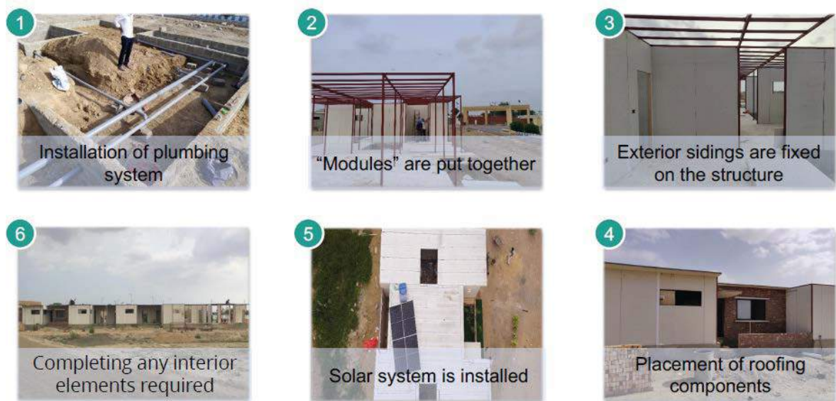
Figure 5: Assembly of a ModulusTech affordable home
