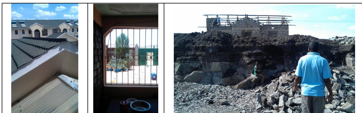
Images 3 (Left to Right): (L) New lightweight sheeting is replacing heavier clay tiles and the need for heavier trusses in wood or steel. Although smaller sections are still not being used in the understructure. (M) Door and window frames continue to be in steel with bars to safeguard from theft. The need to feel secure forms an important part of the design, construction and operations of buildings. While it may be hard to persuade people to do away with these entirely some robust alternatives are available such as the green hedge fencing seen all across Nairobi which is extremely difficult to cut through. (R) Another key problem with Nairobi sites is the enormous expenditure involved in preparing sites with black cotton soil (BCS) and its disposal once the construction has started. Preparing ground and foundations can sometimes cost more than the superstructure, in many instances up to 40-50% of the overall construction cost (excluding siteworks). Mounds of BCS can be found all over Nairobi just abandoned or awaiting suitable disposal. On smaller sites, the stone underneath can be utilized for foundation and walling material with potential savings for construction purposes saving both fuel and transport costs.
