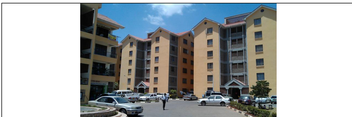
Image 5: Zoning regulations can impact on housing affordability Car parking space is mandatory on some sites even if not entirely necessary to its users. Such rules make it difficult to maximize development potential of land making development costlier. On the other hand it is easily observable that nearly all affordable dwellings have some measure of commercial uses built into them (above left side of image). The same is true for a large number of multi-storey rental housing seen across Nairobi. They all have shops at the ground floor that enhances the return from the building. This practice is in line with good practice elsewhere globally [See Max Lock Centre (London), 'Good Practice in Core Area Development']
