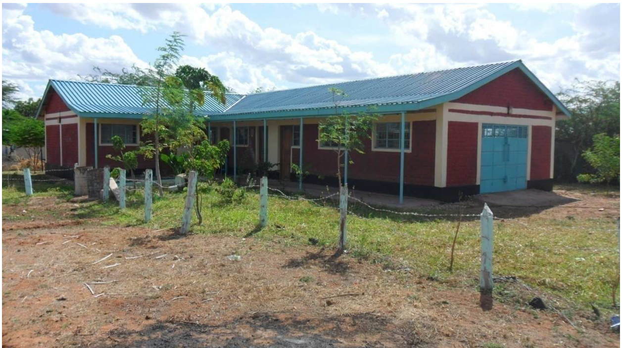
Samples of Houses Constructed using ABM&Ts.
