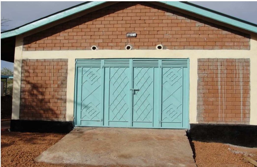
Samples of Houses Constructed using ABM&Ts.
