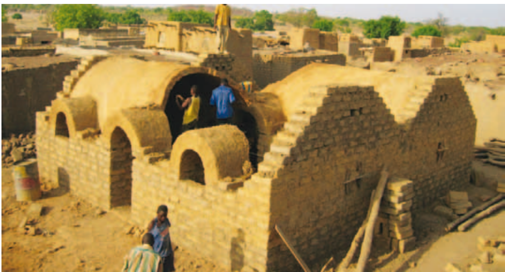
Construction of a two-vault Nubian Vault house, Burkina Faso. © AVN.
