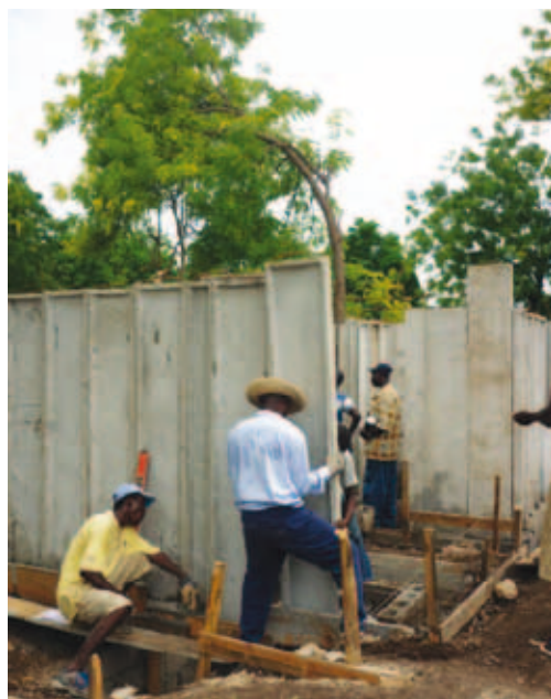
One mason and three helpers assemble the house. © Ecosur.
