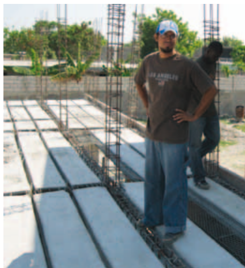
Using ferro-cement panels as floorslab in a conventional building. © Ecosur.
