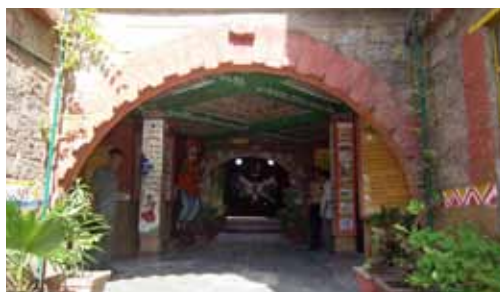
Bhoomiheen camp. A school project built with the same technologies. © Anangpur Building Centre.
