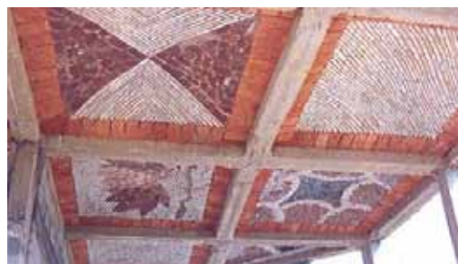
Funicular shells as flooring and roofing constructed using waste stone. © Anangpur Building Centre.
