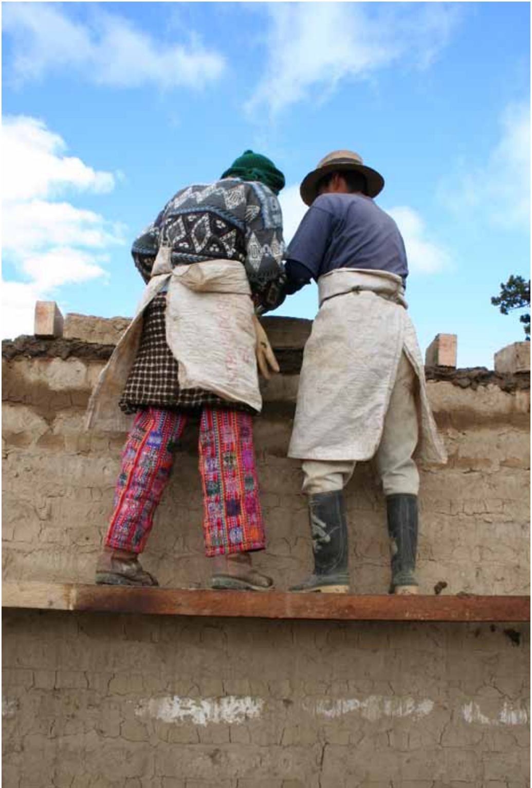
Adobe construction in Guatemala. © Matthew French, UN-Habitat.
