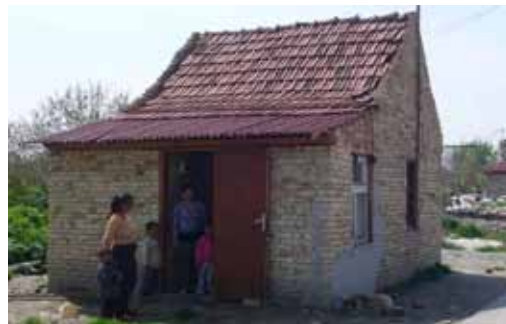
Roma house in Djurdjevo after upgrading. © Daniel Wyss, Skat Consulting Ltd.
