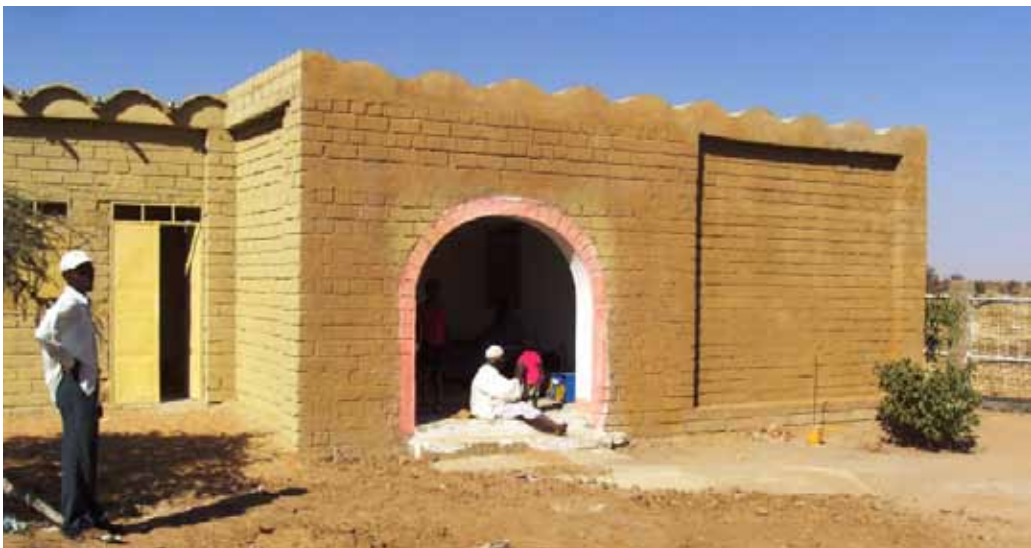
A house built by SSB for disabled headed IDP house-hold in Sakali Area - Southern Darfur in 2010. © UN-Habitat.
