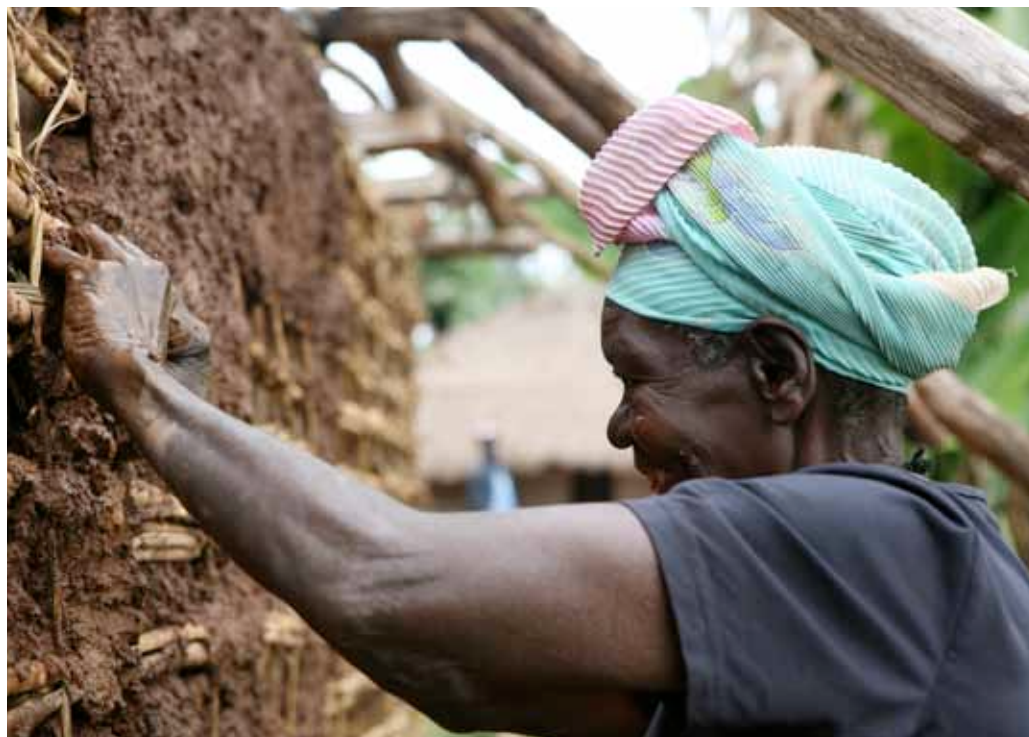
A woman constructing a mud house in Mahagi DRC. © Zahra Moloo, IRIN.
