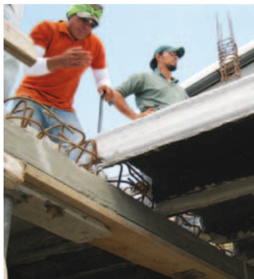
Placing the horizontal panels with the help of a chain-pulley. © Ecosur.
