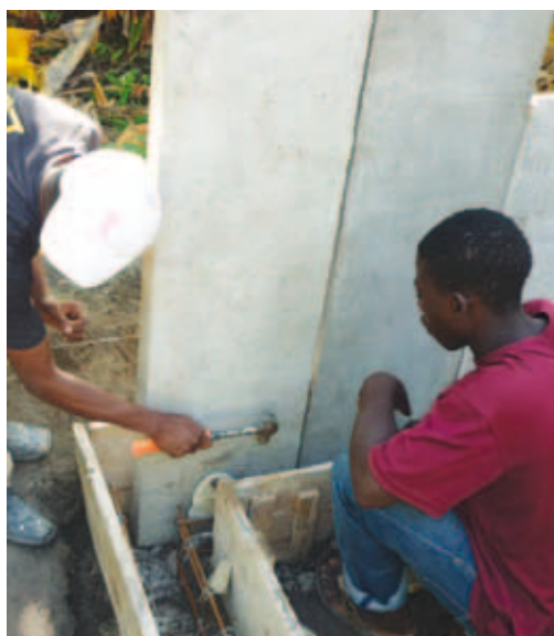
The panels are placed and then concreted into the ringbeam. © Ecosur.
