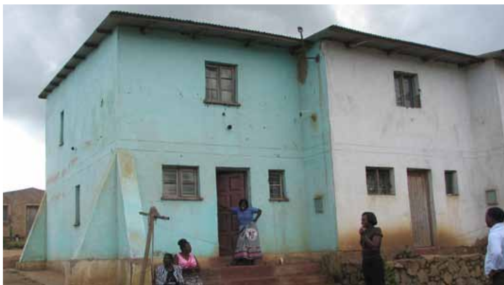
A house constructed by the Women Savings Group in Malawi Peoples Federation. © Graham Tipple, UN-Habitat.
