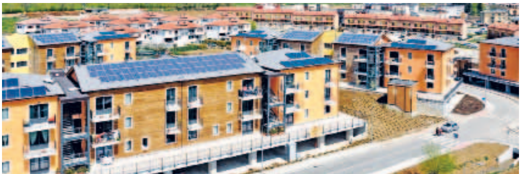
The C.A.S.E. project: Multistorey buildings in Preturo. Installation of photovoltaic modules in combination with solar panels on south facing roofing. © by kind permission of Enerpoint S.P.A ( www.enerpoint.it ).
