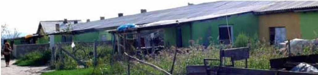
Roma Slum “Bangladesh” in Novi Sad (above: before, below: after the upgrading). © Daniel Wyss, Skat Consulting Ltd.
