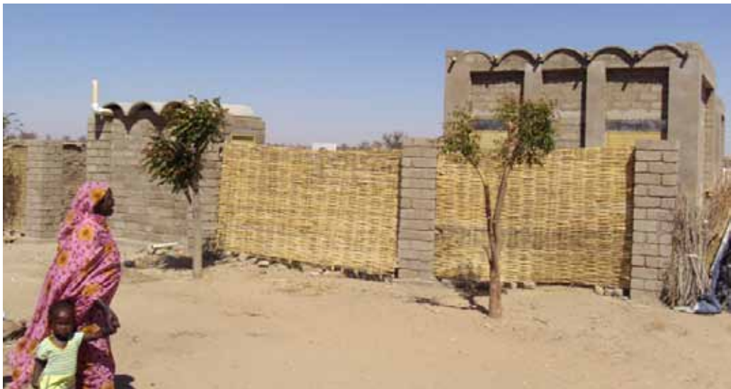
A housing unit built by SSB for a vulnerable IDP family in Sakali - Southern Darfur in 2010. © UN-Habitat.
