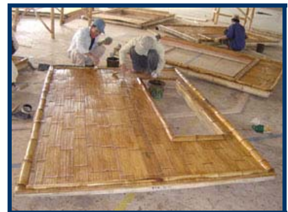
Painting prefabricated door
