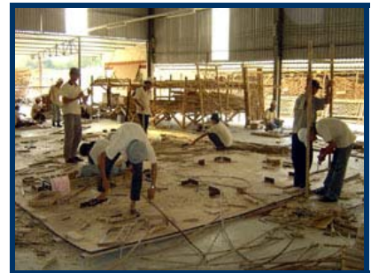
Prefabricated of walls & doors
