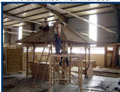
Pre fabricated of tree house
