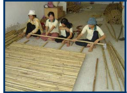
Pre fabrication of bamboo walls
