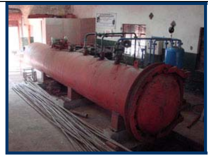
Pressurised bamboo treatment
