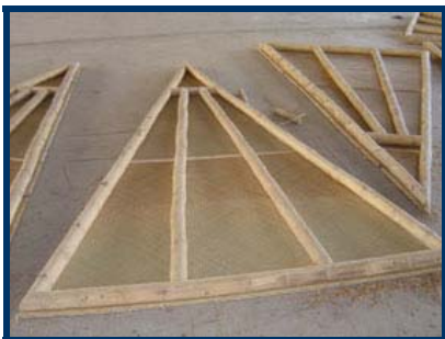
Pre fabricated truss
