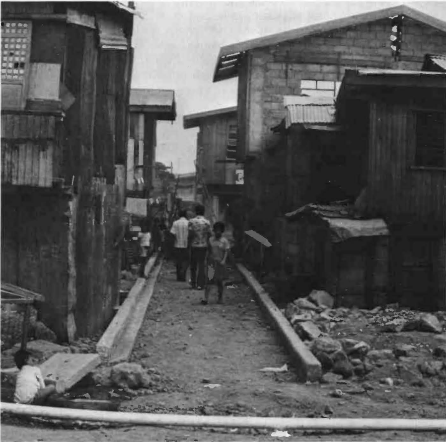
In Tondo, Manila, the existing housing is upgraded and alleys are provided with curbs. The building plots are demarcated for sale.
