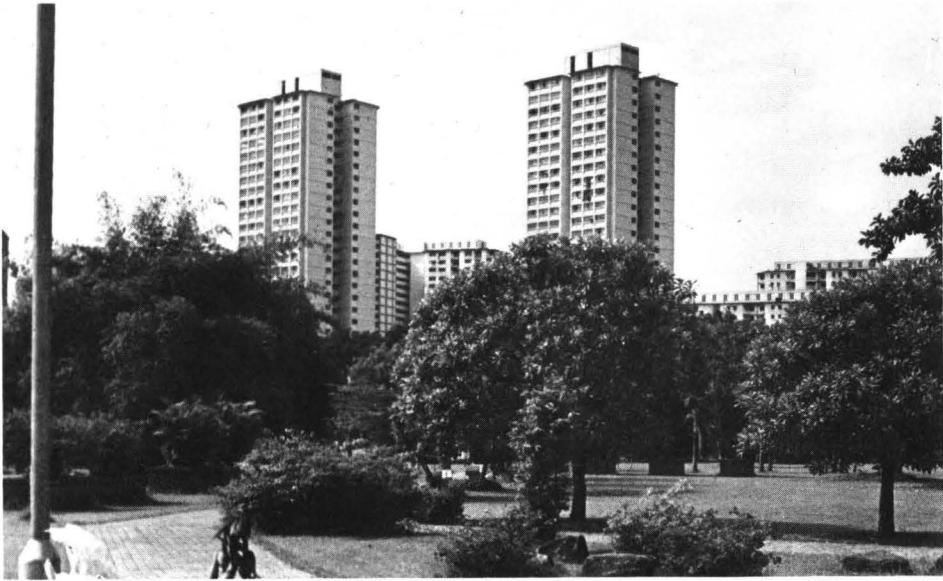
The Bukit Merah Estate in Singapore comprises point-block buildings with 4-room flats.
