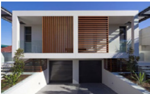
Figure 3-72 Privacy screens can be an integral part of the articulation. Changing the pattern and direction of the screen adds visual interest and asymmetry to the facade.
