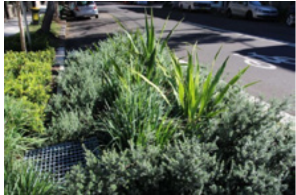
Figure 3-101 Rain gardens integrated into the landscape can filter stormwater
