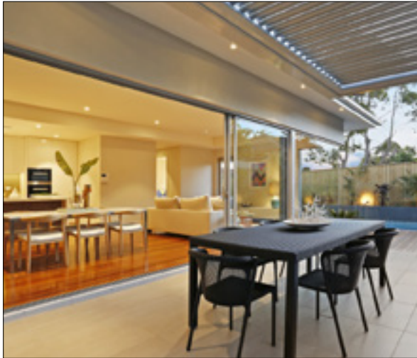
Figure 3-114 A universally designed dwelling provides step free door transitions and level flooring to reduce trip hazards
