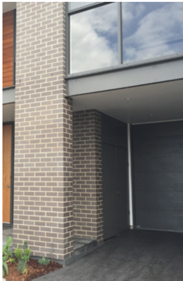
Figure 3-107 Provide bin areas that are screened and incorporated into the landscape or building design
