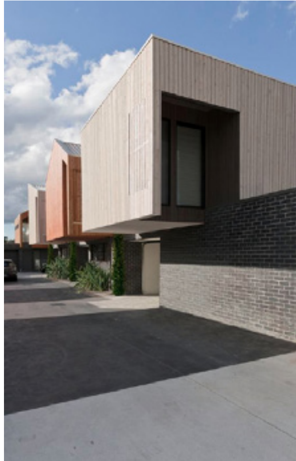
Figure 3-73 A poor acoustic outcome is achieved when driveways are in close proximity to bedrooms and living rooms, and driveways are hard paved reverberating sound.
