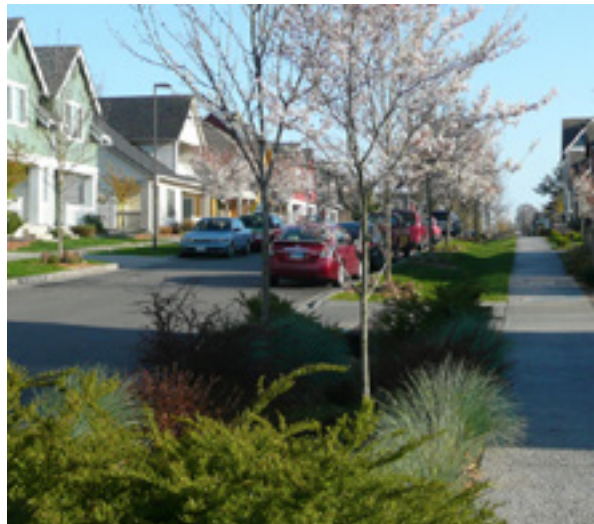
Figure 3-102 Swales can be attractive, and are able to filter and collect the stormwater
