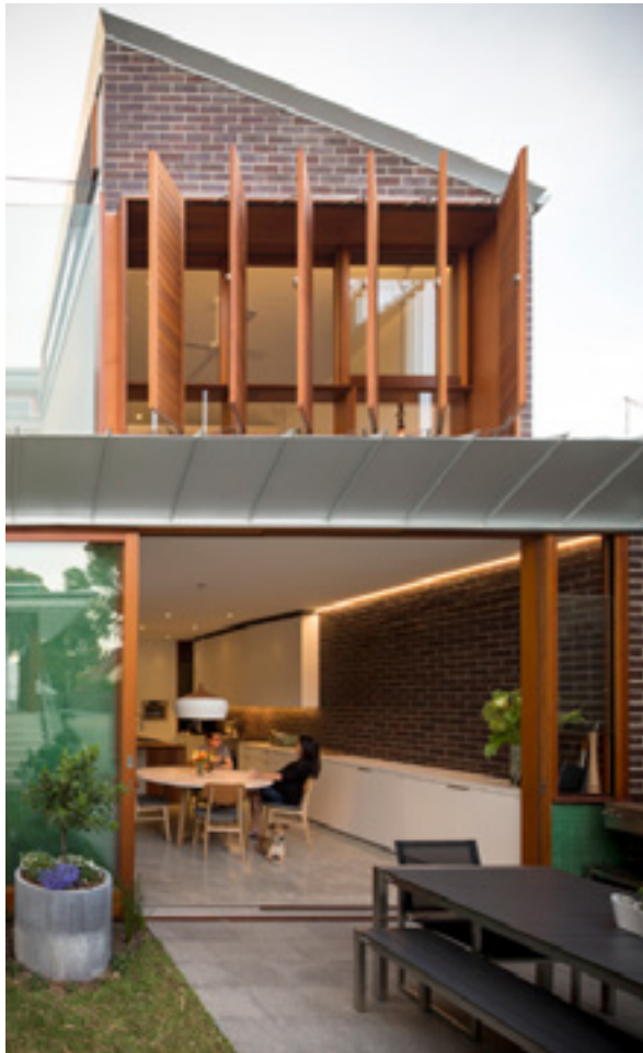
Figure 3-100 Adjustable screens allow control of sunlight
