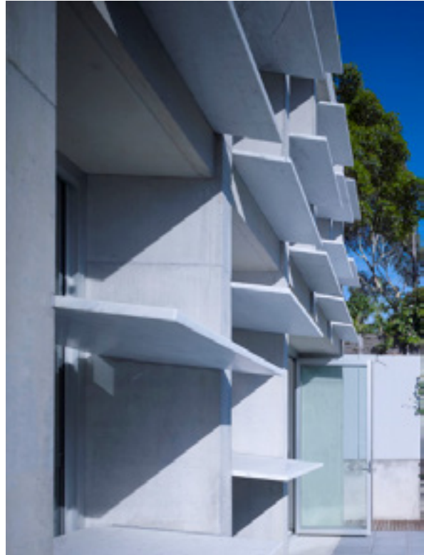
Figure 3-98 Light shelves can reflect sunlight deeper into rooms and provide shade from summer sun
