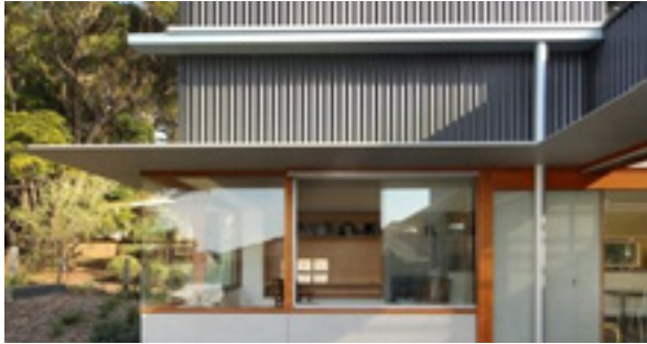
Figure 3-88 Awnings provide shelter and add articulation
