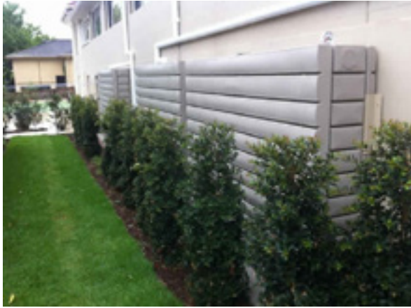
Figure 3-105 Integrate rainwater tanks into the landscape
