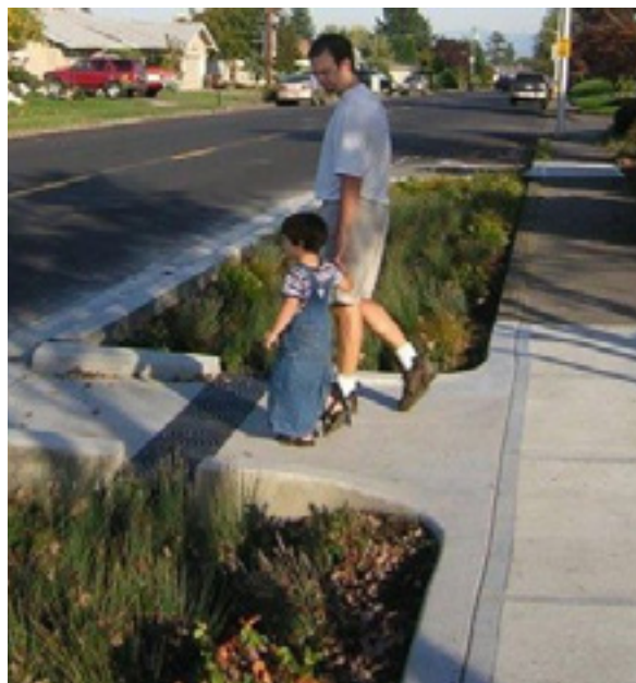
Figure 4-3 Rain gardens treat stormwater from the streets
