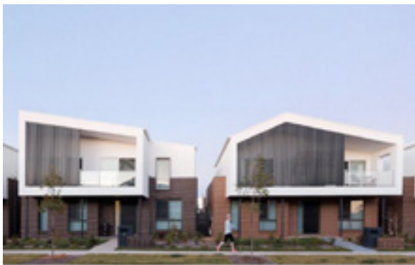
Figure 3-90 The use of screens provides privacy to balconies
