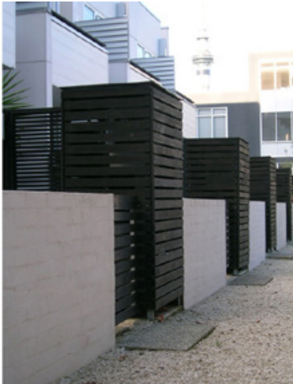
Figure 3-108 Bin areas fronting the street can be designed and incorporated into the building or landscape elements
