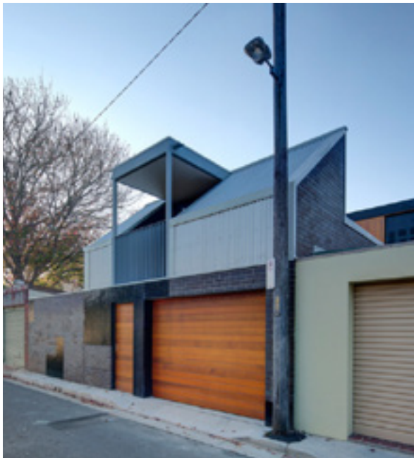
Figure 3-96 Rear outbuildings such as studios should be orientated to the lane to allow for passive surveillance and security
