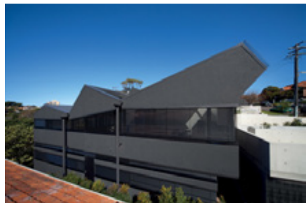
Figure 3-79 Interesting roof forms and integration of privacy and sun control devices to overall building design
