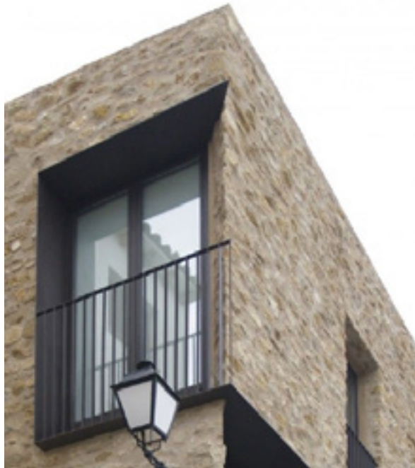
Figure 3-89 Contrast texture with sharply defined openings and fine steel balustrades
