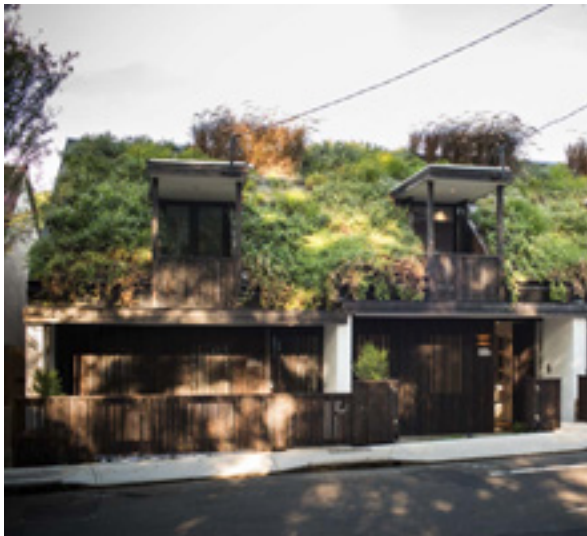
Figure 3-13 Green roof on terraces
