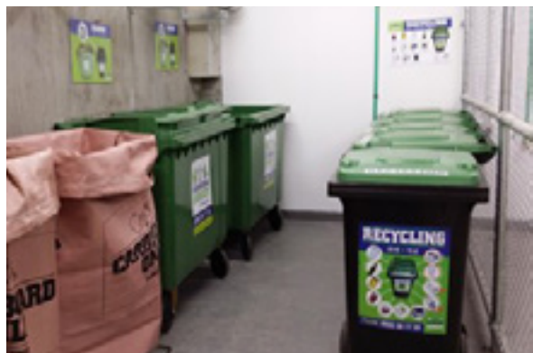
Figure 3-111 Waste and recycling areas should allow for sufficient space to manoeuvre bins and sort waste for recycling
