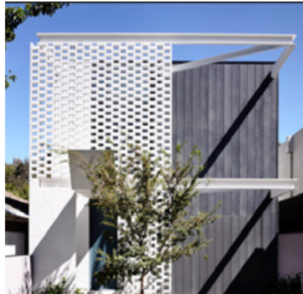
Figure 3-66 Privacy screens are integrated into the facade and provide part of the architectural expression
