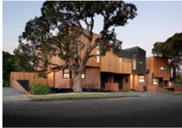
Figure 3-85 Varied building forms and a mixed palette of materials adds interest to the streetscape
