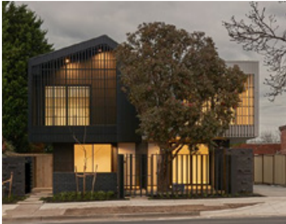
Figure 3-86 Example of transparent fencing landscaping in front setback and asymmetrical facade design
