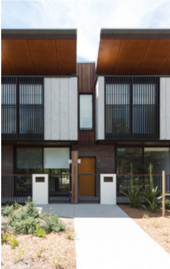
Figure 3-74 Living rooms setback from main circulation spaces by large landscape setback provides privacy
