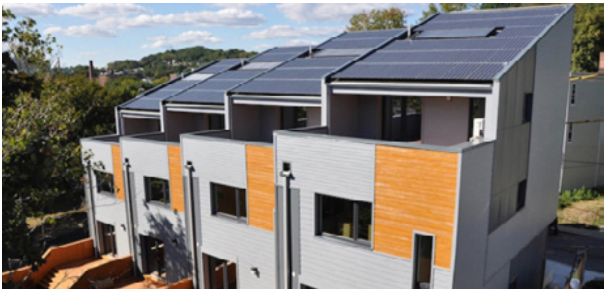
Figure 3-97 Roof mounted photovoltaics should be integrated into the design of the dwelling
