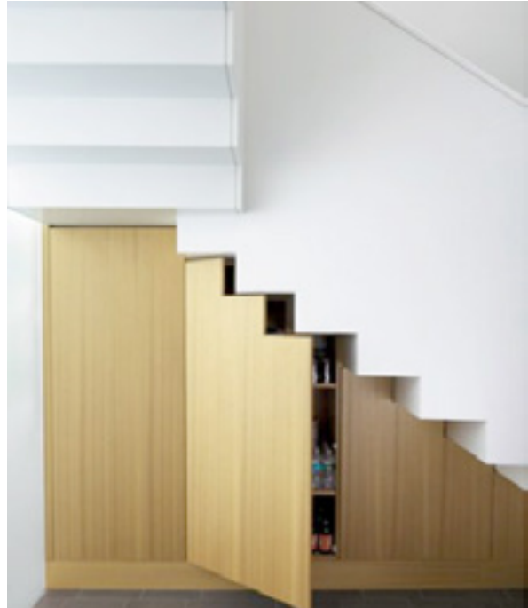
Figure 3-58 Storage space under stairs
