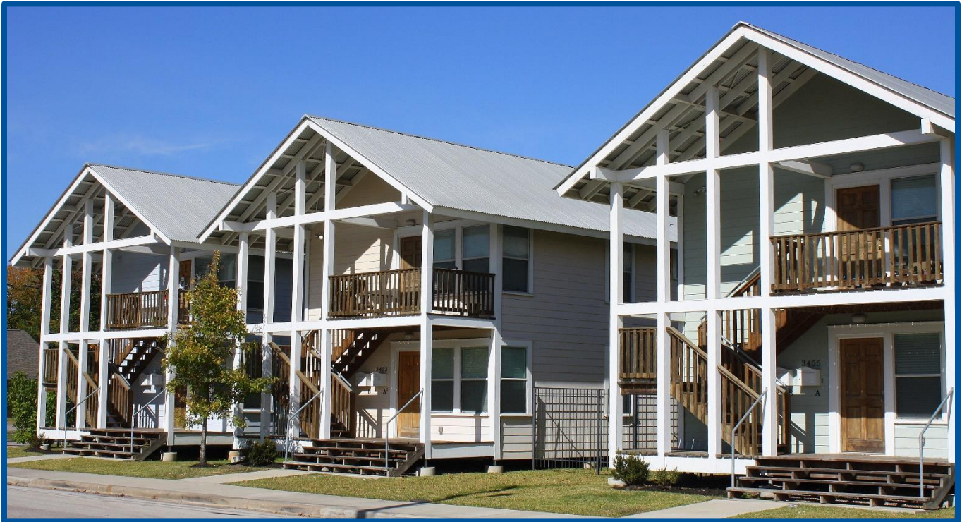
Figure 45: MRA Duplexes Located near Napoleon and Tuam in the Third Ward
