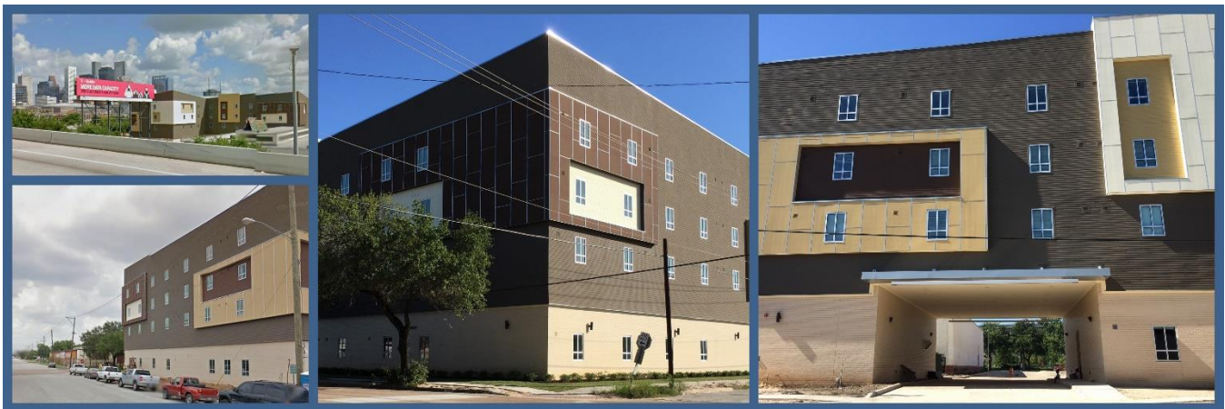
Figure 43: Images of the Newly Constructed Temenos Place II Apartments
