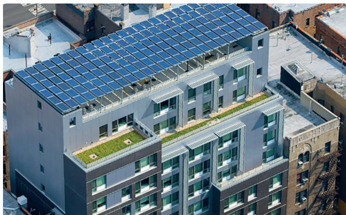
A rooftop solar PV array on a multifamily apartment building in Brooklyn, New York. Photo credit Bright Power, Inc.
