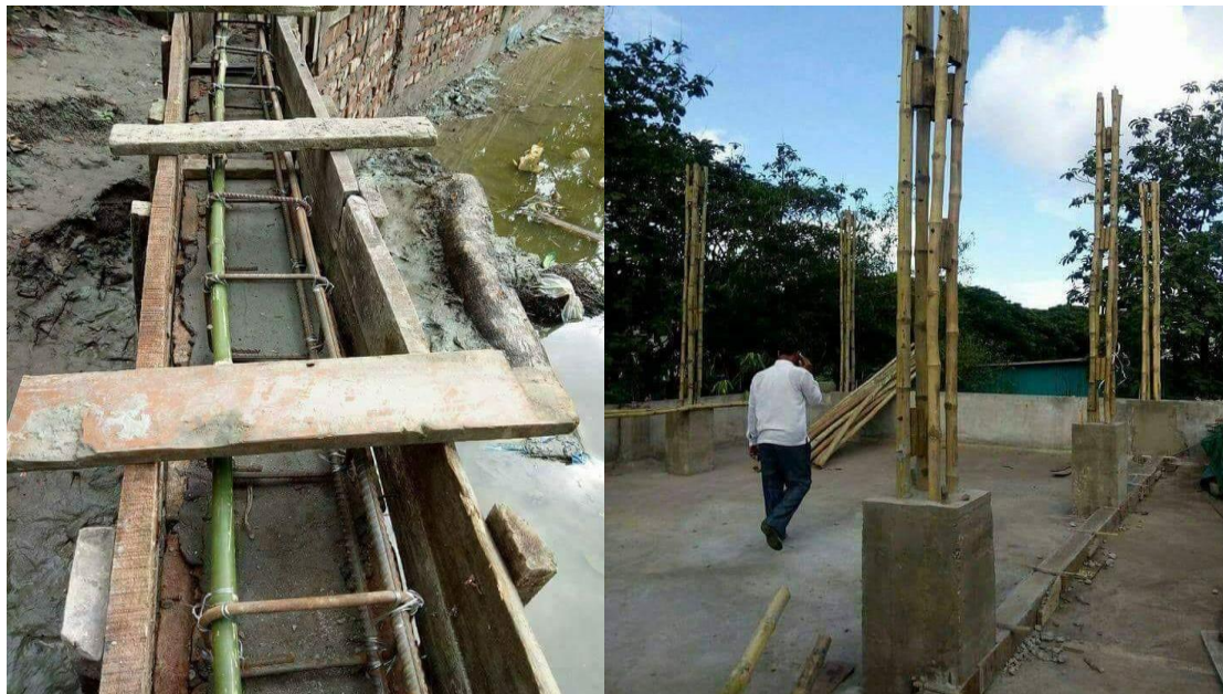
Figure 2. Bamboo used to reinforce concrete in ground beam and columns
