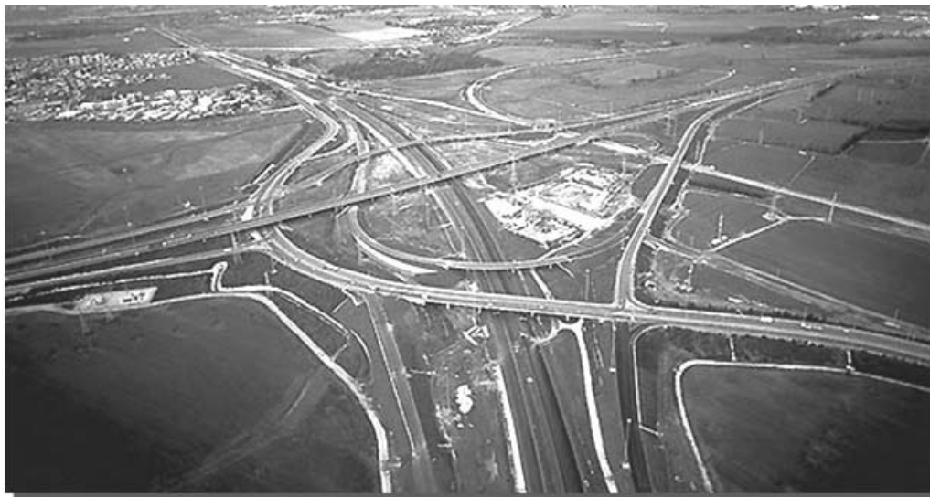
FIGURE 7: A View of Highway 6 in Israel
