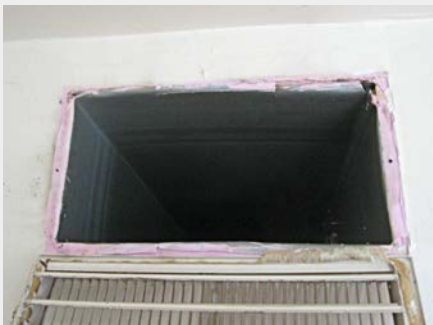
Sealing duct registers and boots to ceilings or floors can dramatically reduce unwanted duct leakage.
