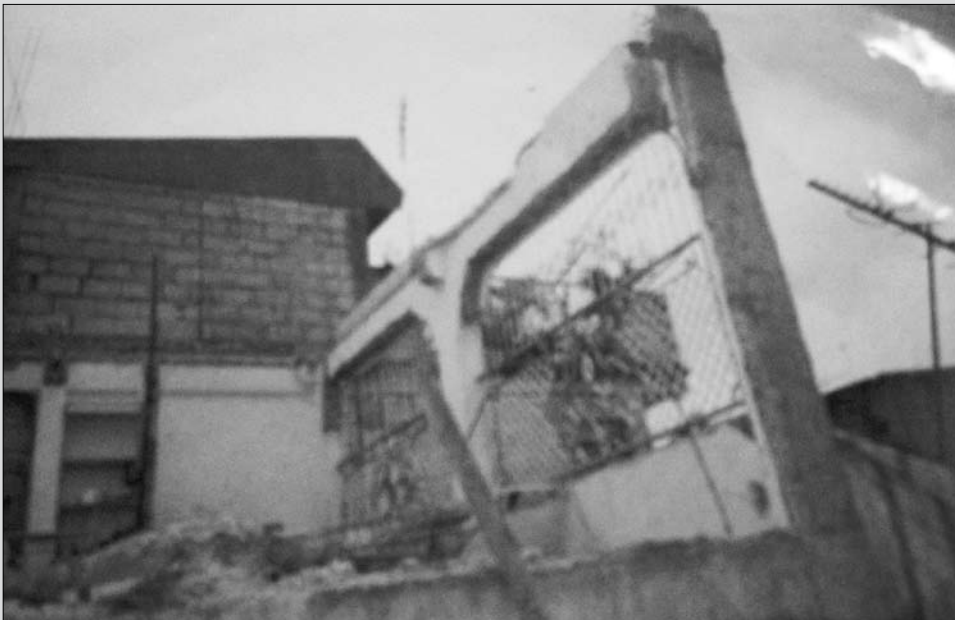
Demolishment of the housing unit of a recalcitrant household © UN-HABITAT
