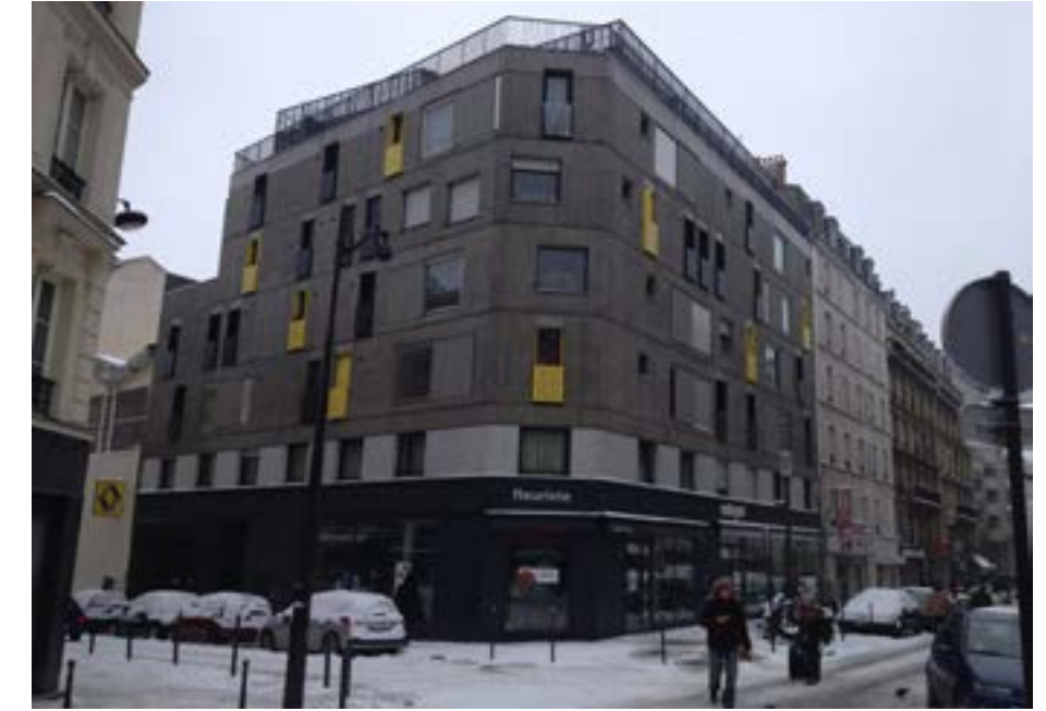
Image 26: New construction for housing
