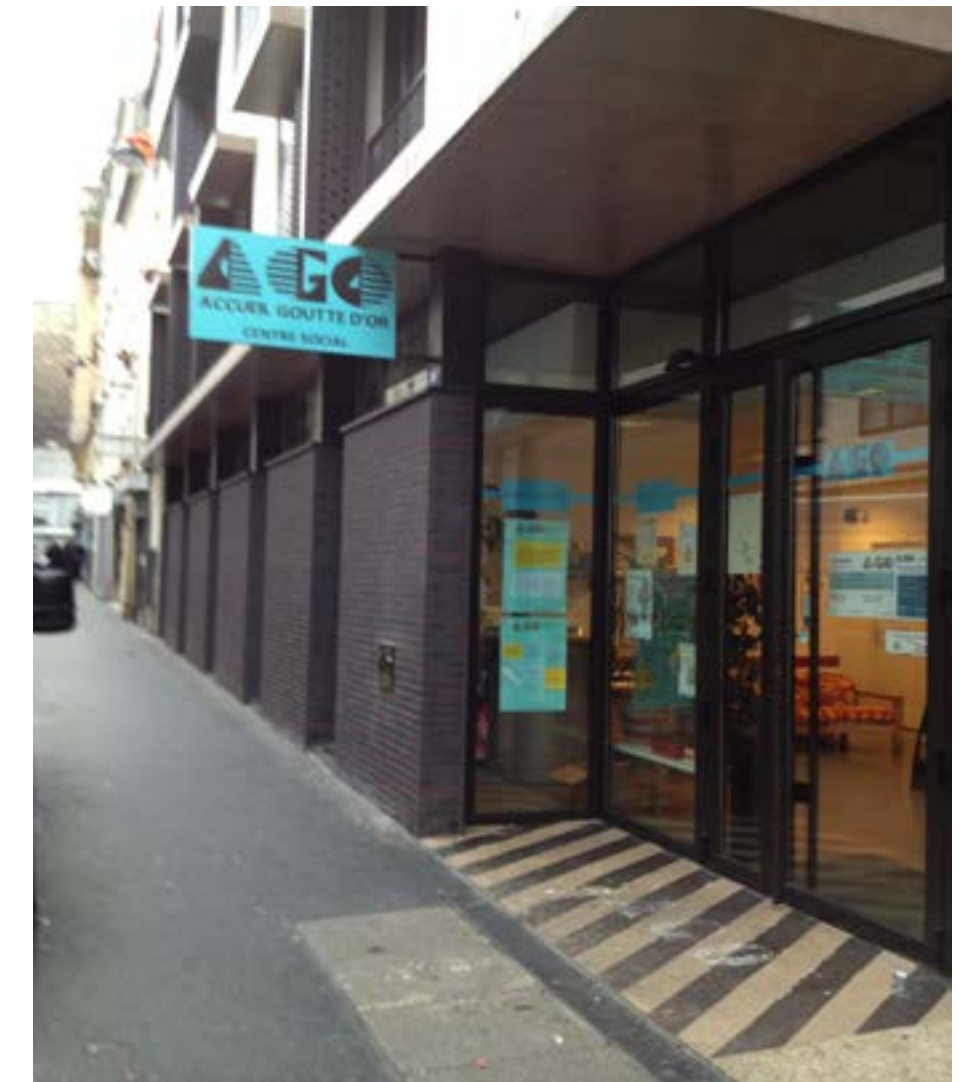
Image 22: Accueil Goutte-D'Or-Centre Social, dedicated to improving economic development in la Goutte d'Or, situated in a newly constructed building
