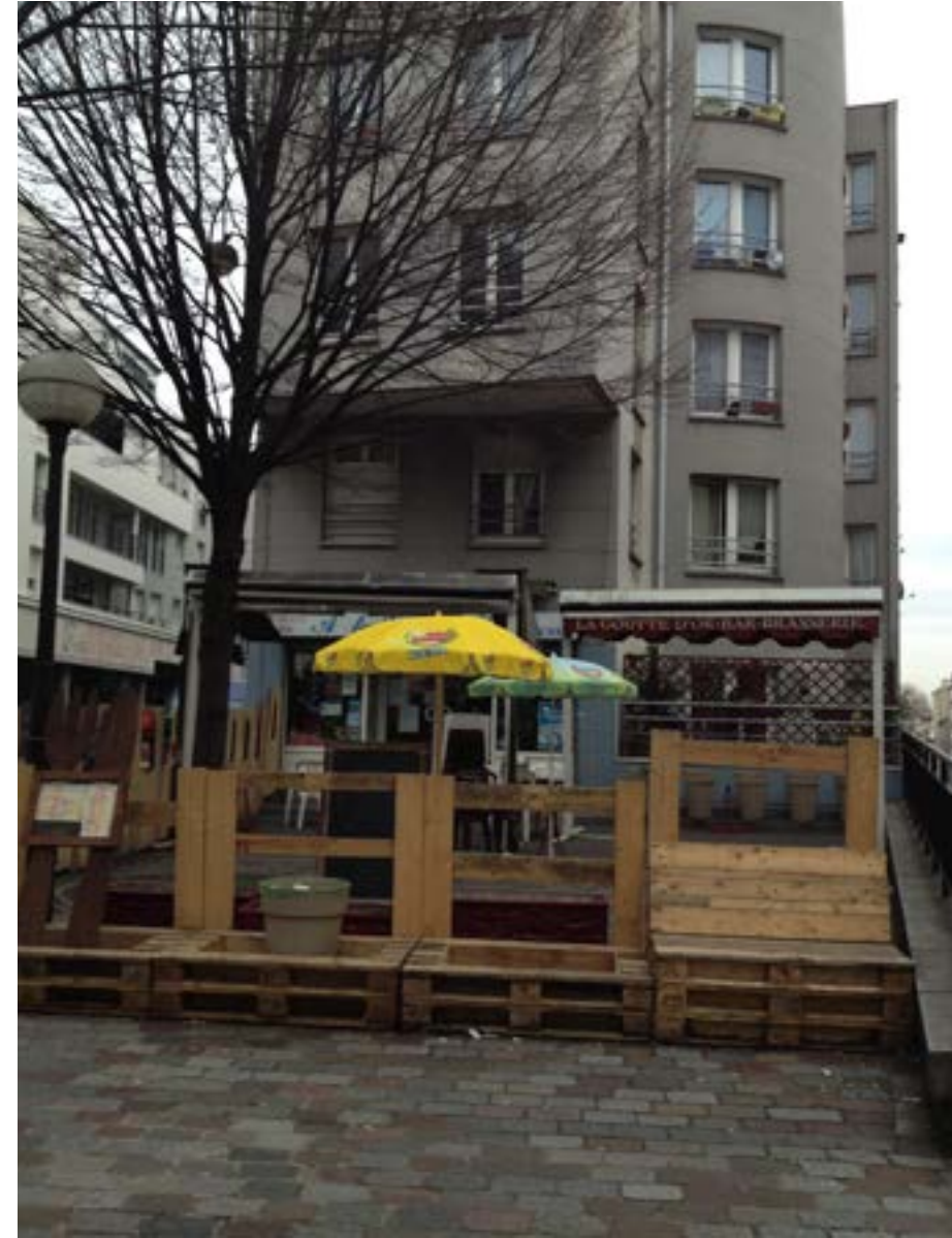
Image 25: Construction underway for a central square with cafe
