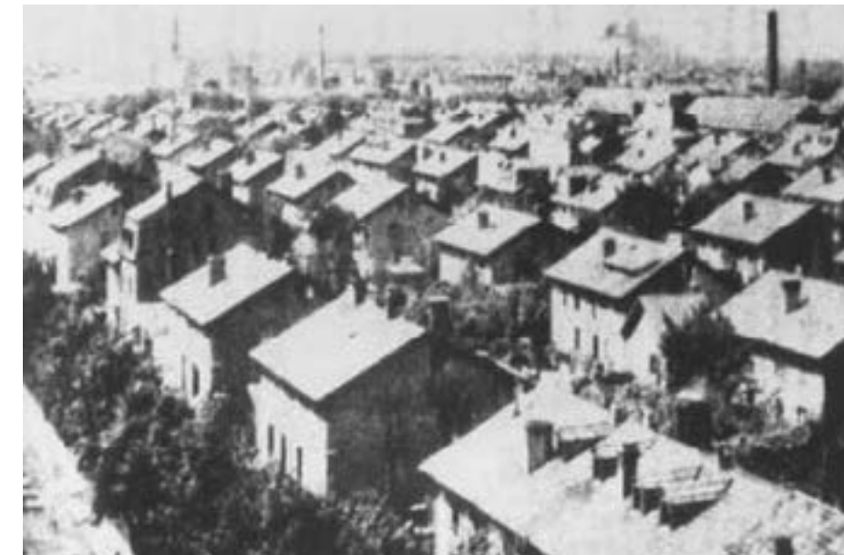
Image 1: Single-family workers housing built by industrialist Jean Dollfus as a model for housing reform Source: http://www.tslr.net/2008/01/reissue-quadruple-houses-in-france.html
