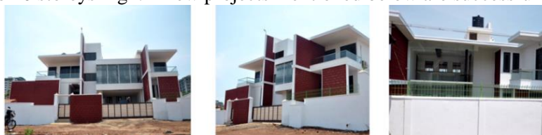
Figure.2. Rapid wall 2 storeyed Residential building at Manipal
