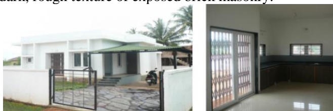
Figure.3. Rapid wall Residential building at Mumbai
