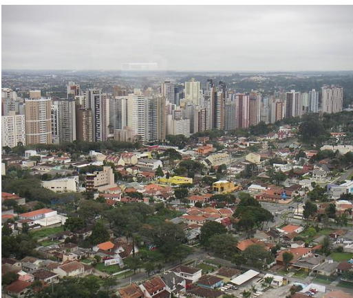
Figure 17: The City of Curitiba (Brazil) is considered an example of “eco-city”, due to its integration between urban development, transportations and public health. Source: https://en.wikipedia.org/wiki/Eco-cities#/media/File:Curitiba_Brazil_Structure.jpg
