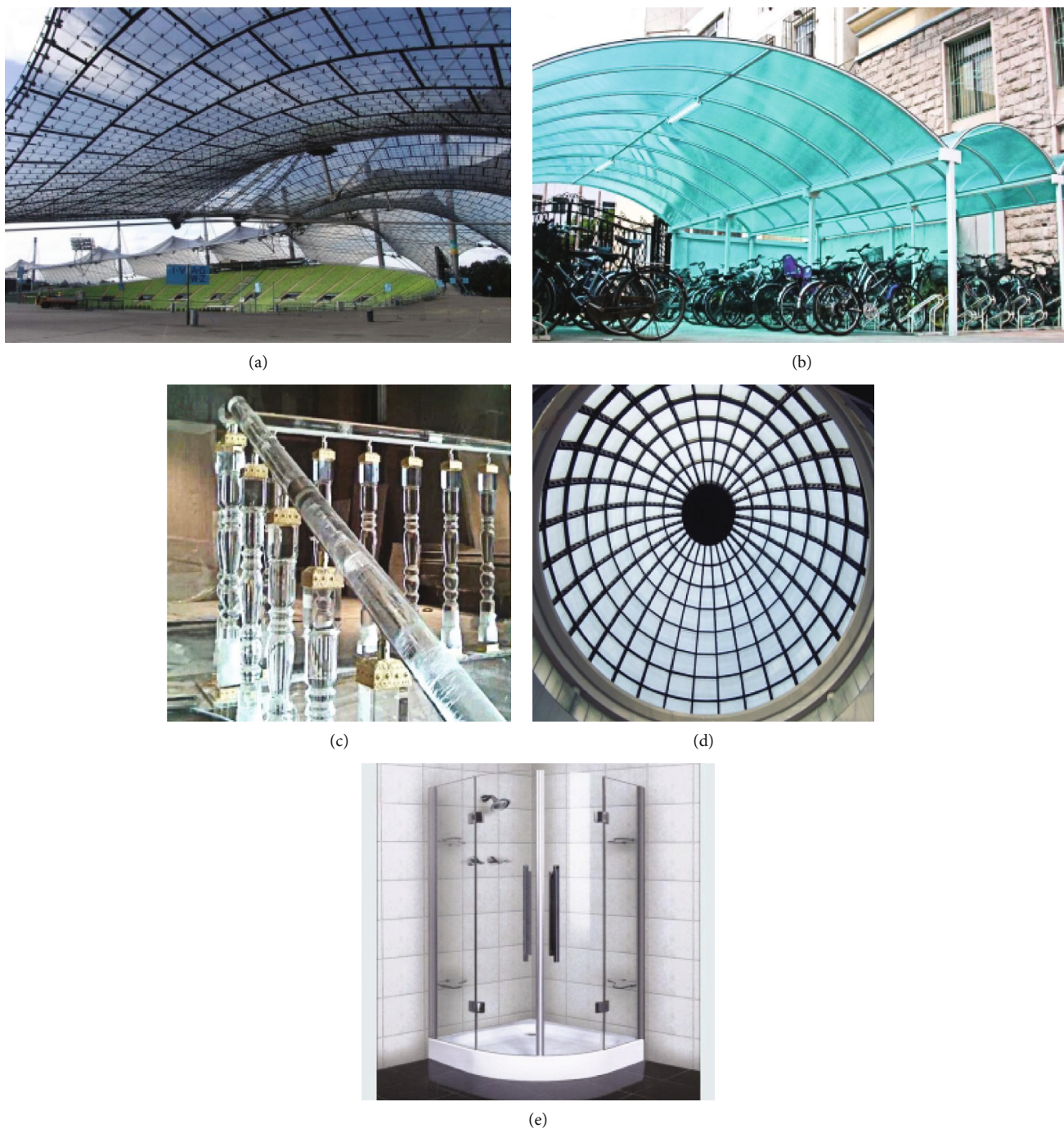
FIGURE 4: Applications of PMMA in construction and buildings. (a) Stadium for the 20th Olympic Games in Munich, Germany. (b) PMMA sun board shed. (c) Cylindrical PMMA stairs. (d) PMMA pyramid of light shade roof skylight glass. (e) Cylindrical PMMA component [71].
