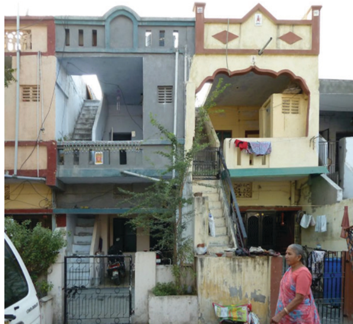
Figure 4: Vernacular style housing in Ahmedabad is no longer allowed by GDCR-2021
