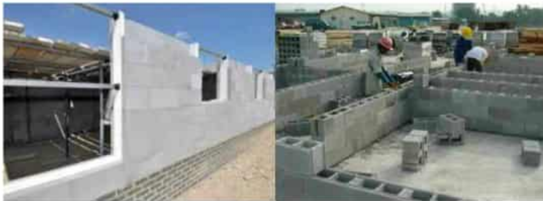
Figure 2.8 Blockwork System
