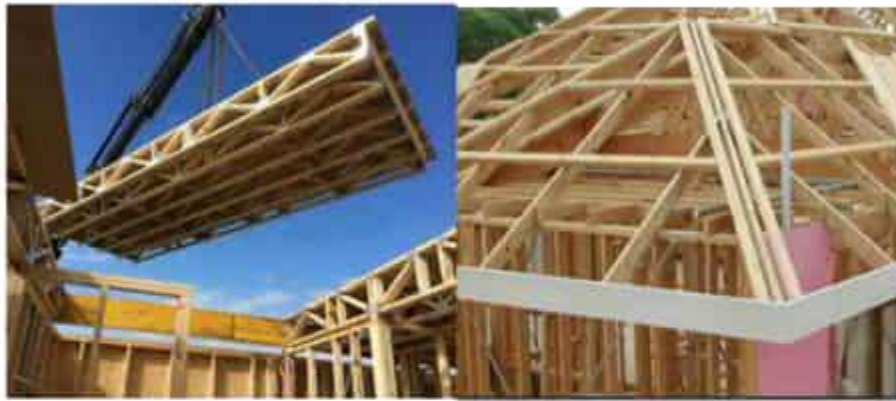
Figure 2.7 Timber Framing System
