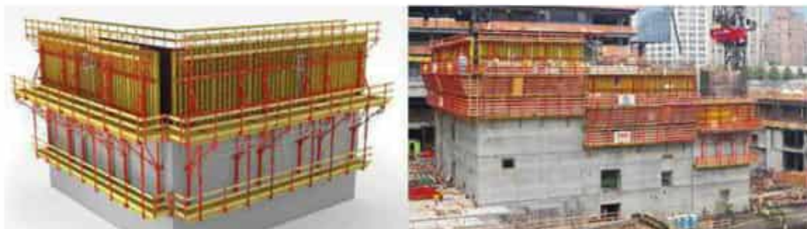
Figure 2.9 Self-Climbing Formwork System
