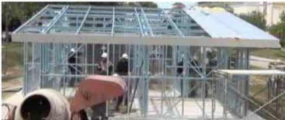
Figure 2.6 Metal Framing System
