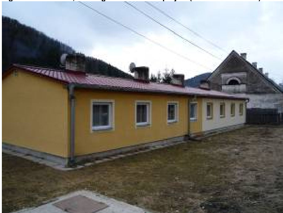
Figure 4 – Vaľkovňa, housing built within the project (view from the road)
