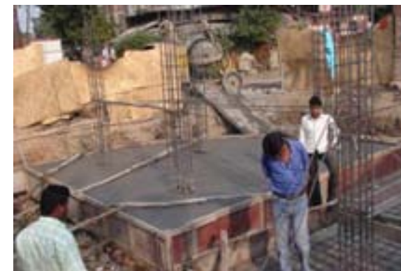
Construction begins on a redeveloped housing unit in Nagpur.
