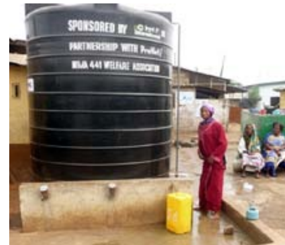
A water kiosk in Ayidiki provides residents with access to clean water.
