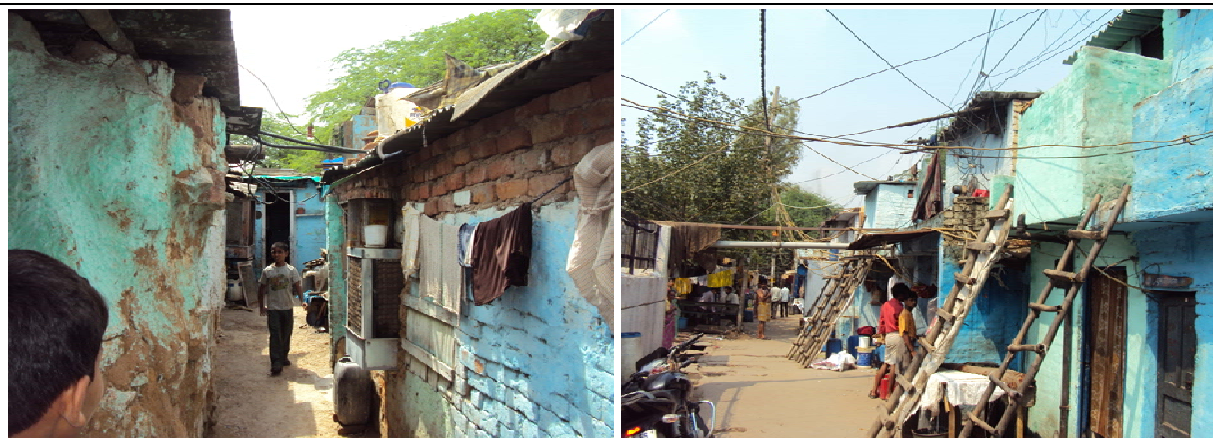
FIGURE 5.3: A SEMI PUCCA DWELLING WITH COOLER FITTED IN WALL (LEFT) AND A MULTISTORIED PUCCA SLUM DWELLING (RIGHT)
