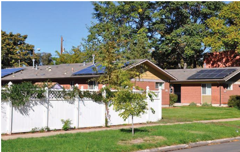
NE Denver Housing Center PV Installation, NREL
