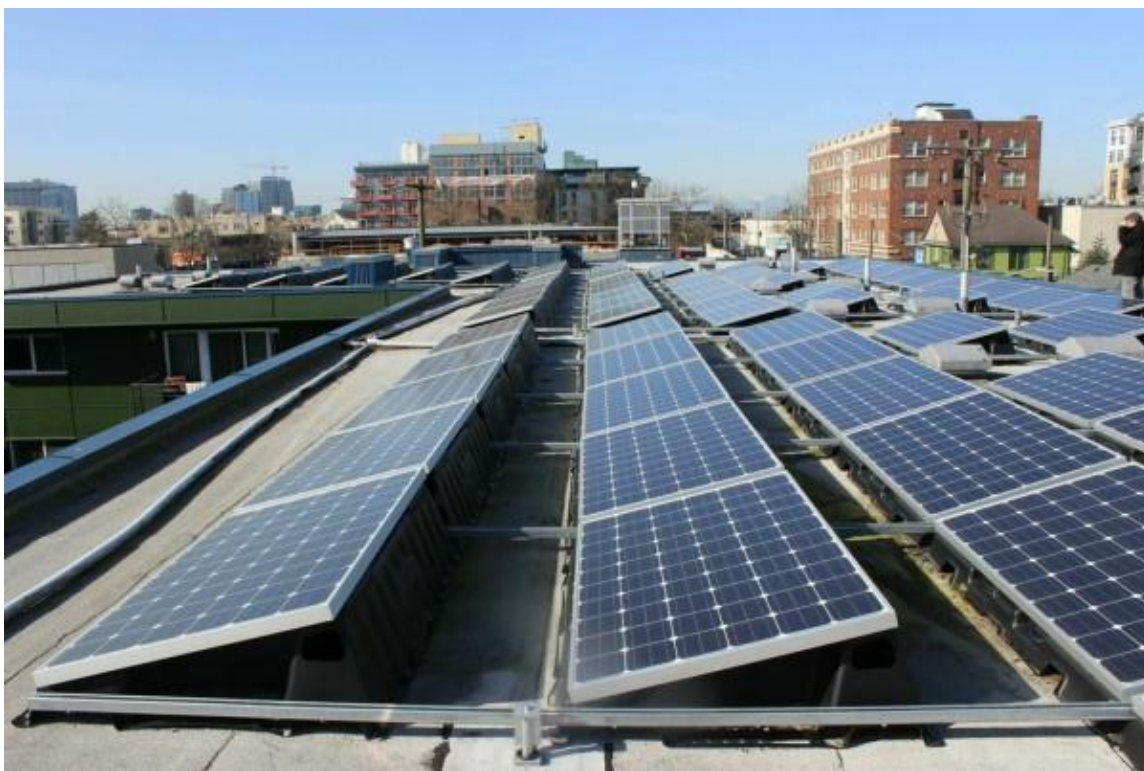
Installation on Capitol Hill Housing's Holiday House
