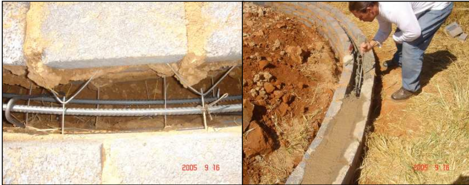
Figure 6.7 – Placing of Foundation Reinforcing & Concrete
