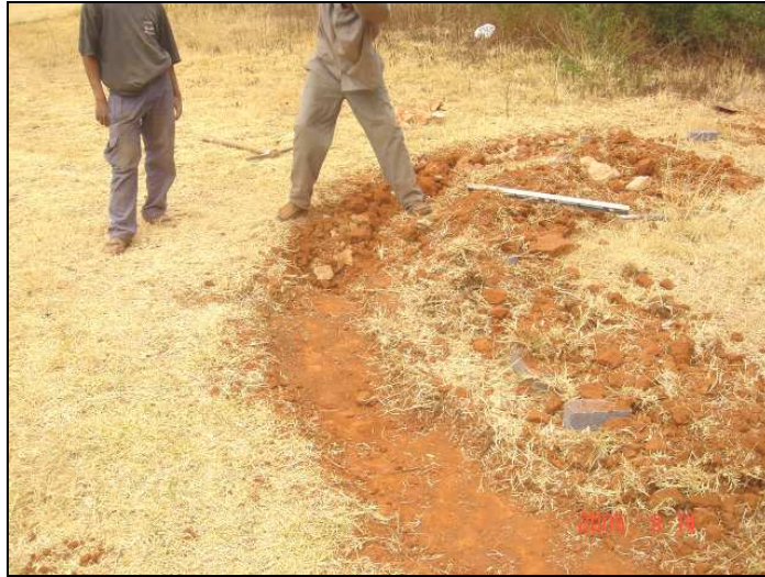
Figure 6.5 – Digging the Foundation
