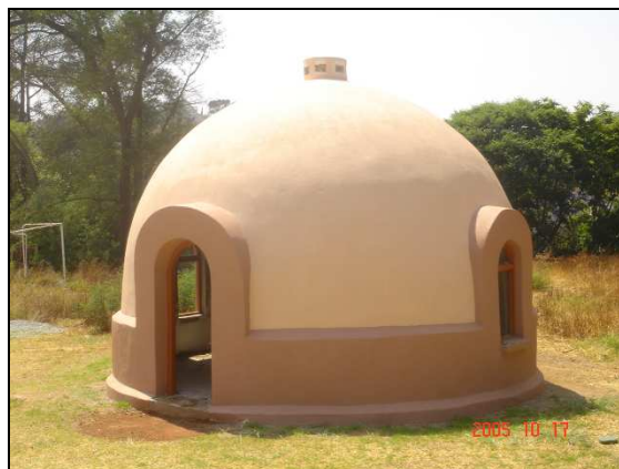
Figure 6.17 – The Completed 28m 2 (301 ft 2 ) Dome
