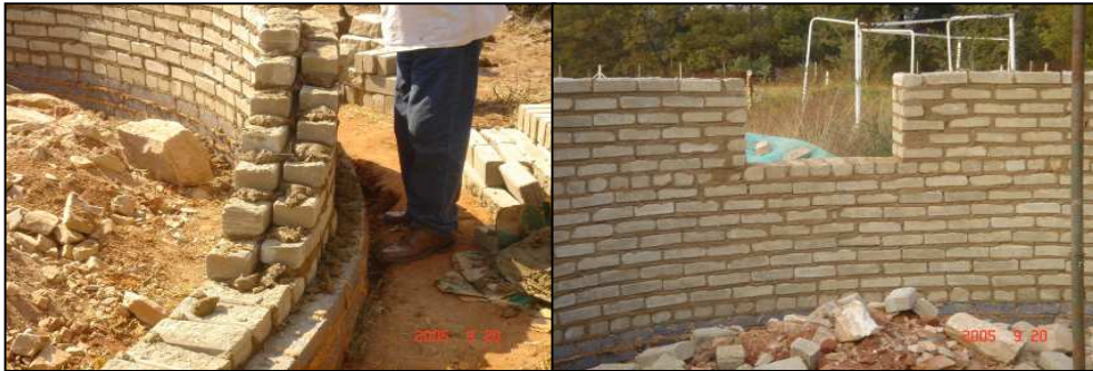
Figure 6.9 – Construction of the Cylinder Wall
