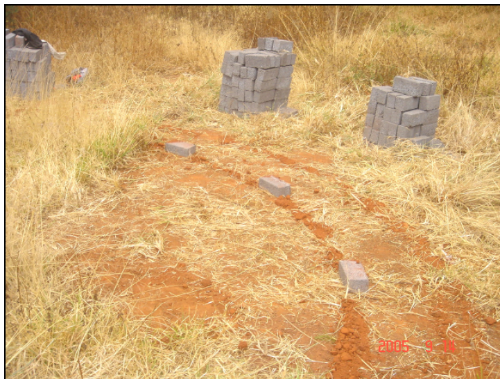
Figure 6.4 – Setting Out of the Foundation
