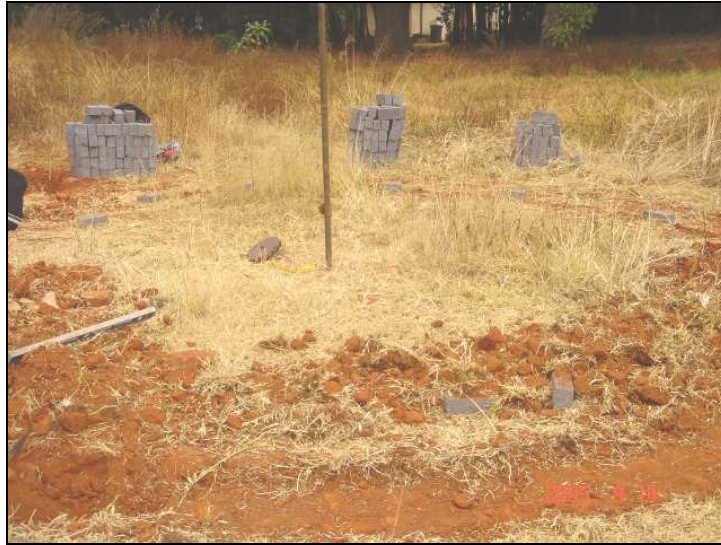
Figure 6.3 – Setting Out Equipment for the Foundation
