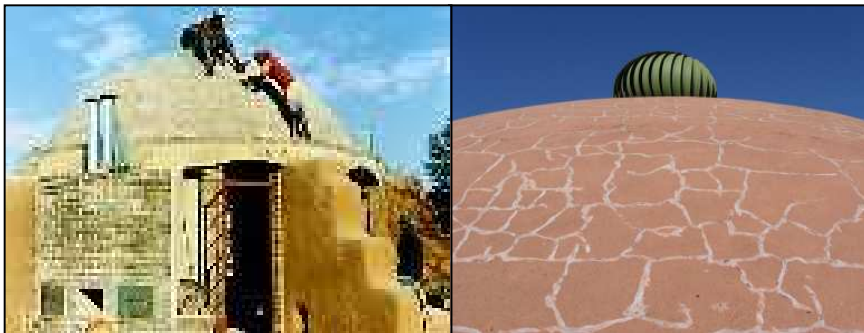
Figure 1.9 – Dome Kitchen – Tlholego Eco-Village
