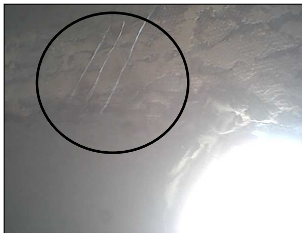
Figure 6.15 – Wire Wrapping around Door Opening
