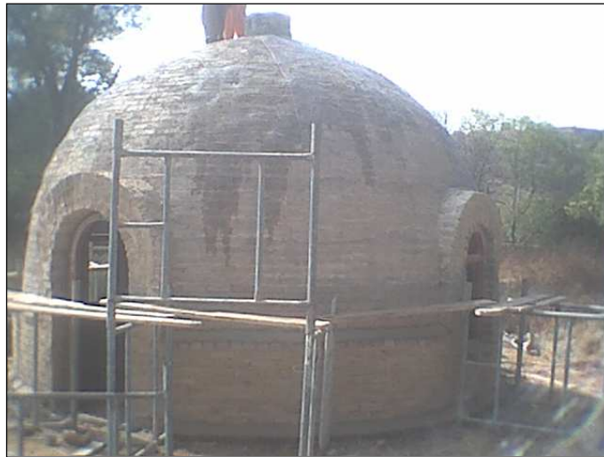
Figure 6.14 – Un-plastered Dome
