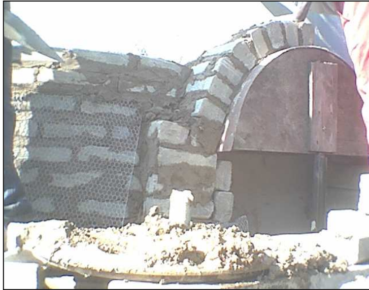
Figure 6.12 – Construction of the Arches
