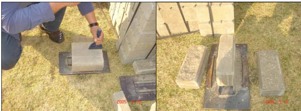
Figure 6.8 – Splitting the Splitter Blocks
