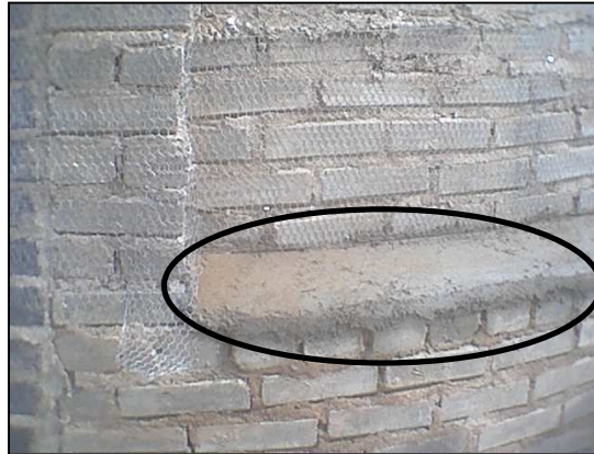
Figure 5.10 – Final Structure - Concrete Lintel
