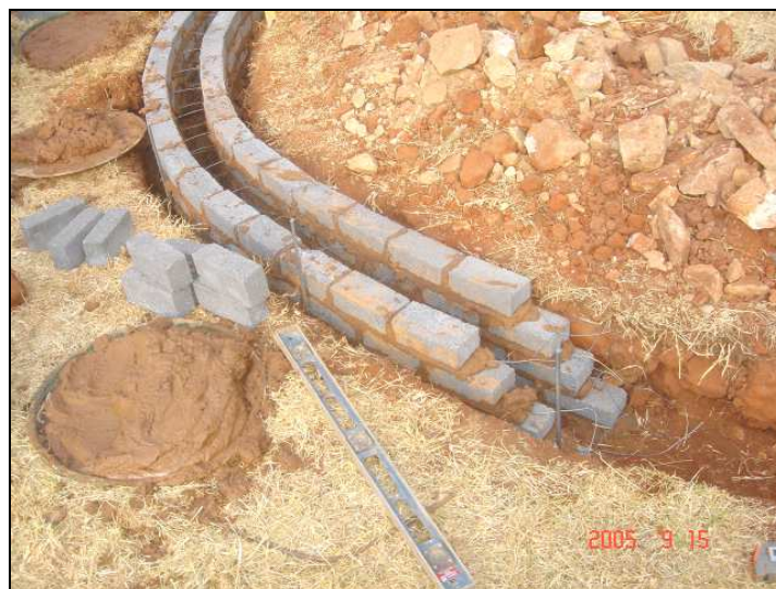
Figure 6.6 – Short Foundation Walls
