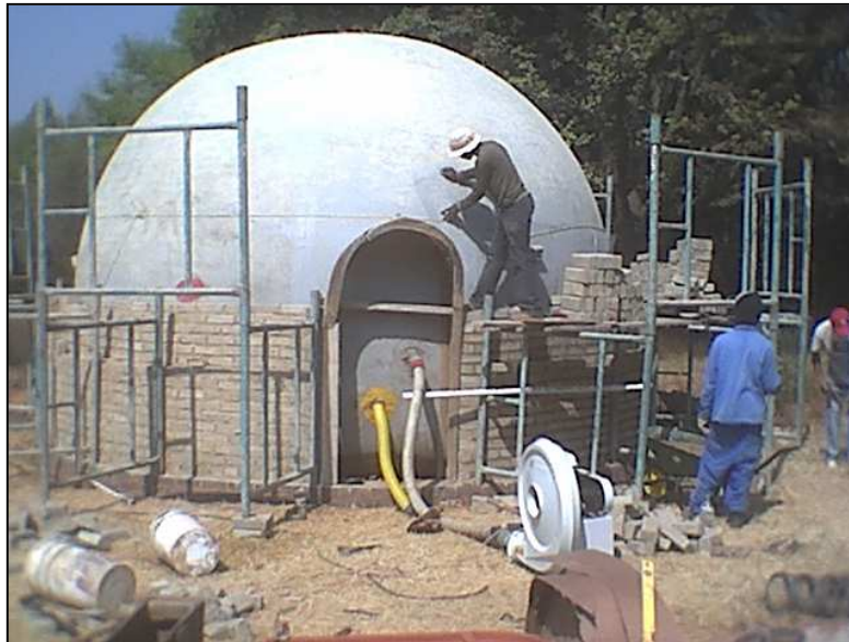
Figure 6.10 – The Inflatable Formwork
