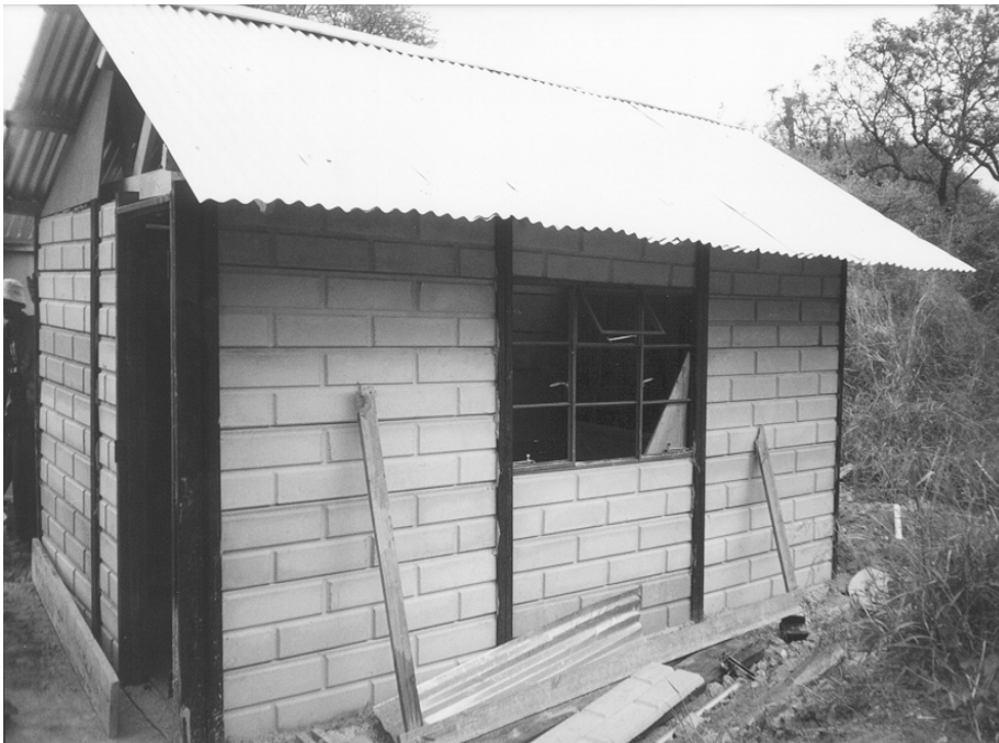
Figure A1: Construction stages of Precast Structure: a) Steel columns; b) Panels, doorframes etc.; c) “Wall plate”; d) Roofing
