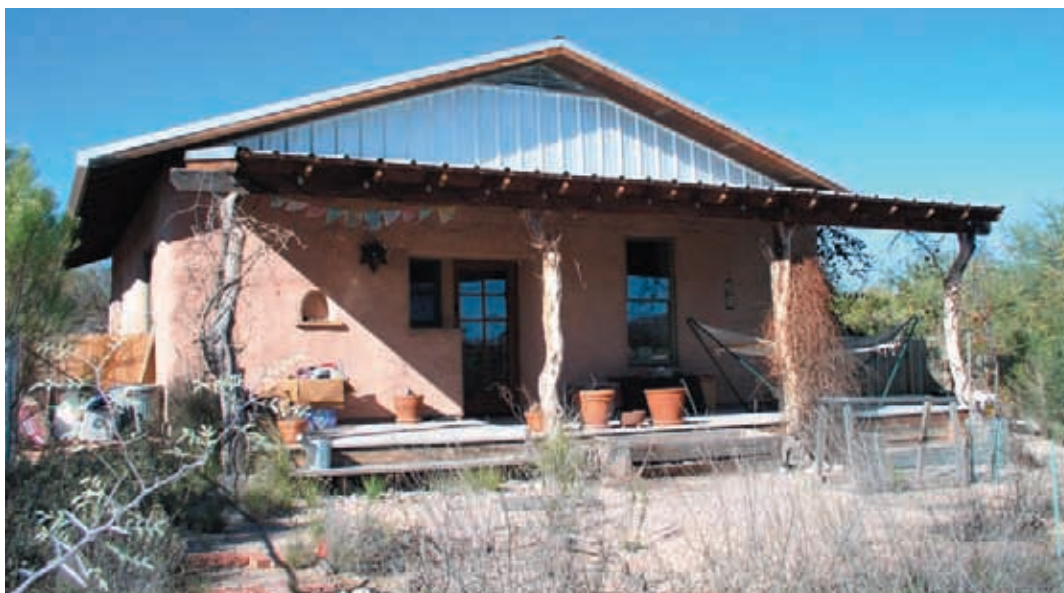
Tucson, AZ: The finished house has an east-facing porch, a sheltered transition from the interior to the desert environment. Earth plaster stabilized with lime and mesquite porch posts from the site demonstrate the integration of regional materials. Deep overhanging eaves provide shade and protect walls from rainfall. Photo: B. Vint
