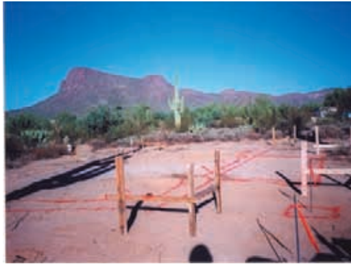
1 Foundation staked and laid out w/ spraypaint.
