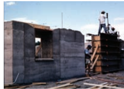
6 Forms built to create voids for windows/ doors.
