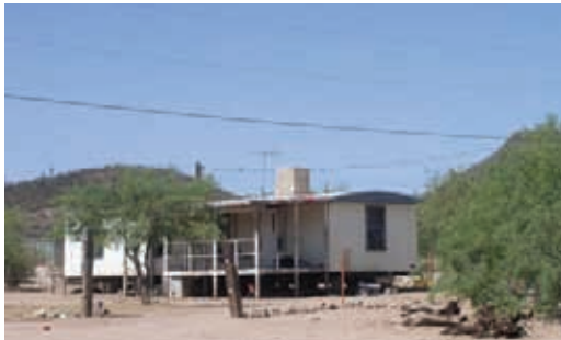
San Xavier District Tobono O'odham Nation, Tucson. The mobile home has little thermal insulation and no thermal mass, so that it becomes super-heated in the summer. Note evaporative cooler ("swamp box") on roof. Photo: B. Vint
