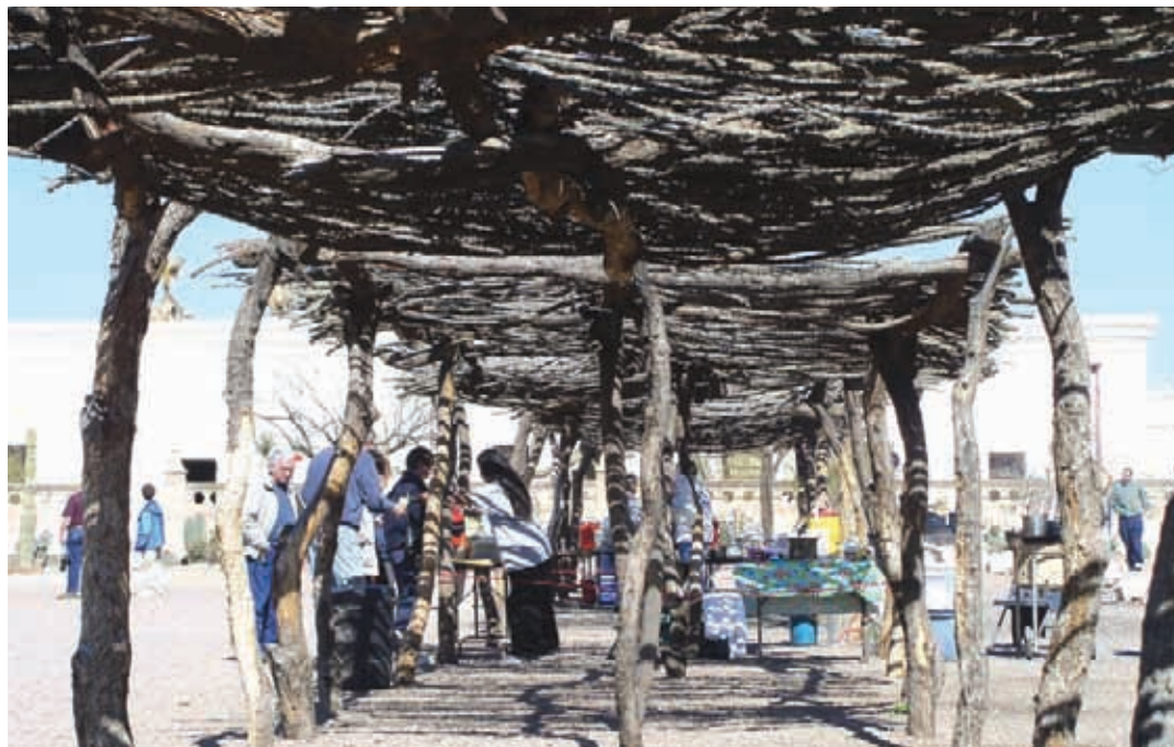
Tobono O'odham wa:tbo (ramada) built of mesquite posts and ocotillo cactus stalks. The shade structure captures the essence of desert architecture. Photo: B. Vint
