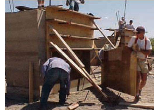
3 Removal of forms.
