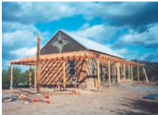
7 metal roofing added and porches framed
