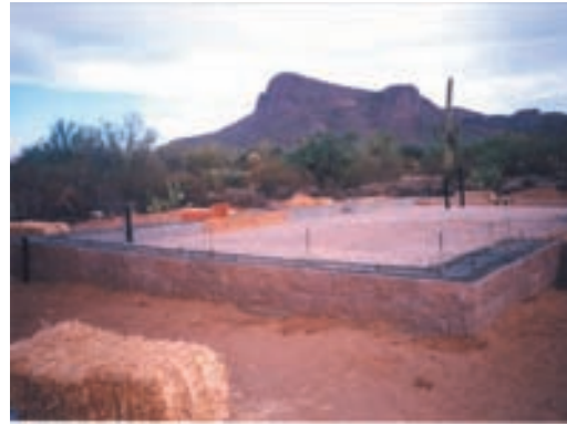
2 Concrete footing poured and block stem wall built.
