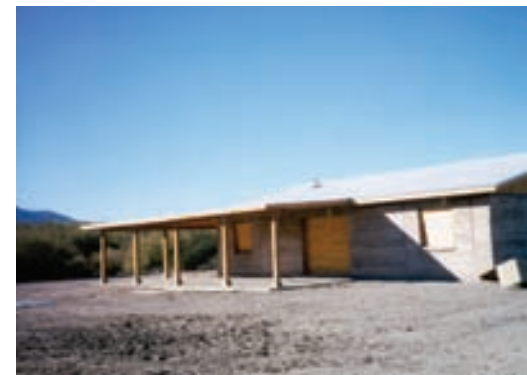
9 Final earthen house before windows and doors.
