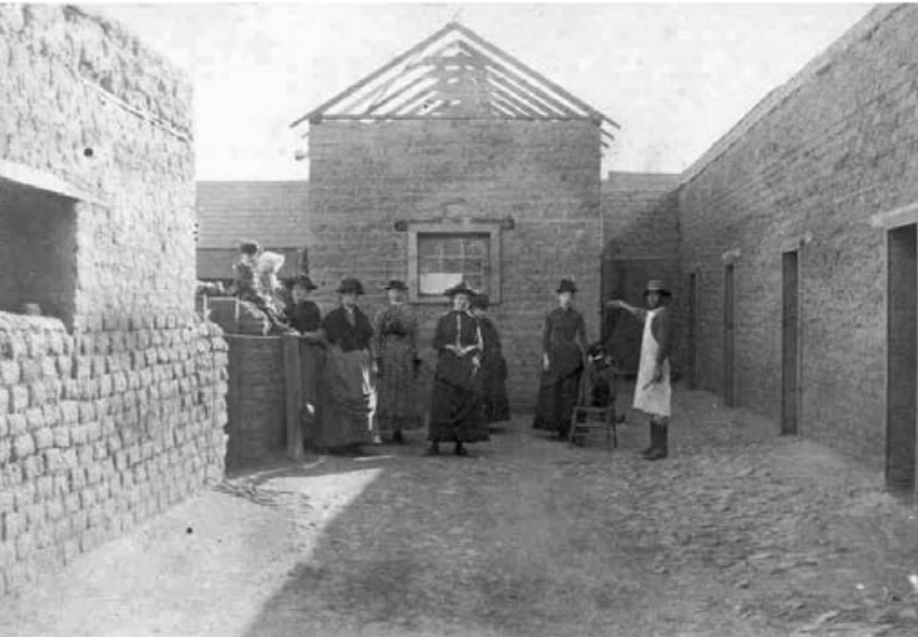
Sheltered outdoor space of the Empire Ranch. Note gabled roof framing in progress over original adobe parapets. Photo courtesy of Laura Vail Ingram, Empire Ranch Foundation
