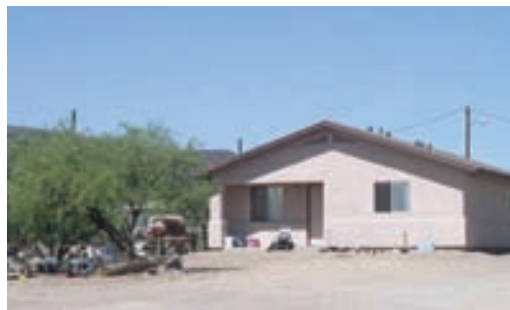
Conventional frame & stucco affordable housing at San Xavier District. Note the thin walls, which are unable to moderate the heat and glare of the desert sun. This type of house requires air conditioning to remain comfortable, resulting in high utility bills for families who often cannot afford them. Photo: B. Vint
