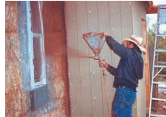
9 clay slip pressure applied before earth plastering
