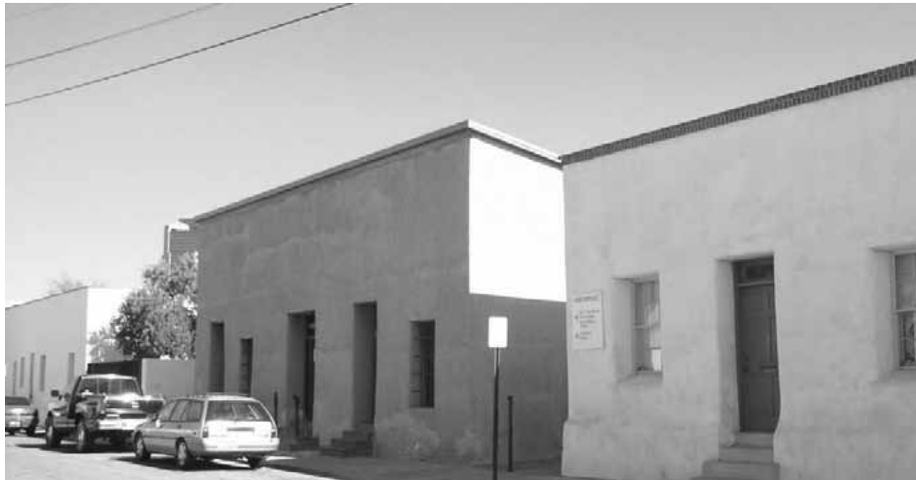
Barrio Viejo, Tucson, AZ: West facade of Casa Carillo.
