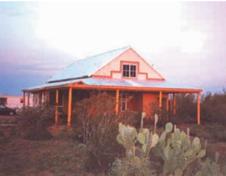
View of completed home from west. Photo: C. Roberts
