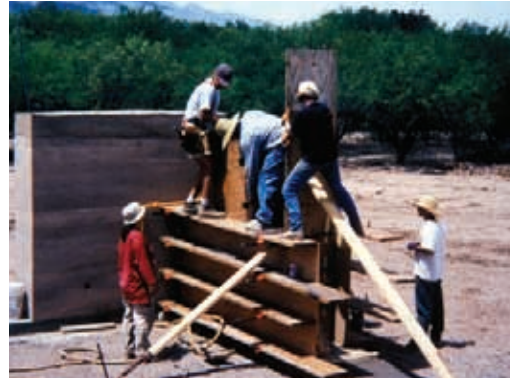
2 Tamping earth within lumber/plywood forms.
