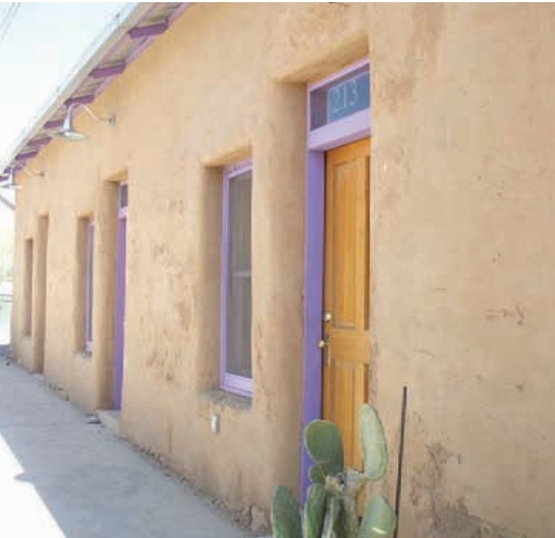
Tucson, AZ: adobe row house with earthen plaster. Photo: C. Neumann
