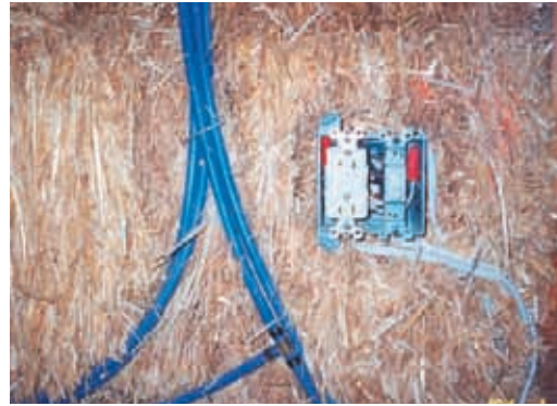
8 electrical conduit integrated with bales
