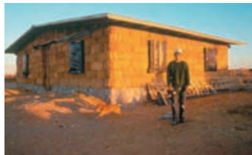
The straw bale house of José Luis before exterior plastering. Photo: C. Waneke
