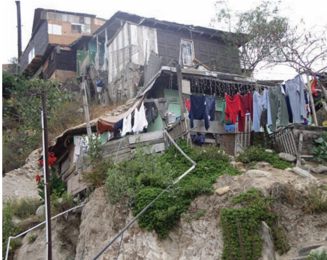
Colonia in Tijuana. The houses of paracaidistas (squatters) are built on marginal land at the edge of town, hilly, inaccessible and hard to build on. Shacks evolve by piecemeal replacement with permanent materials (cinder block and concrete). Gradually the colonias become permanent neighborhoods, as electricity and roads are added. Photo: A. Vint
