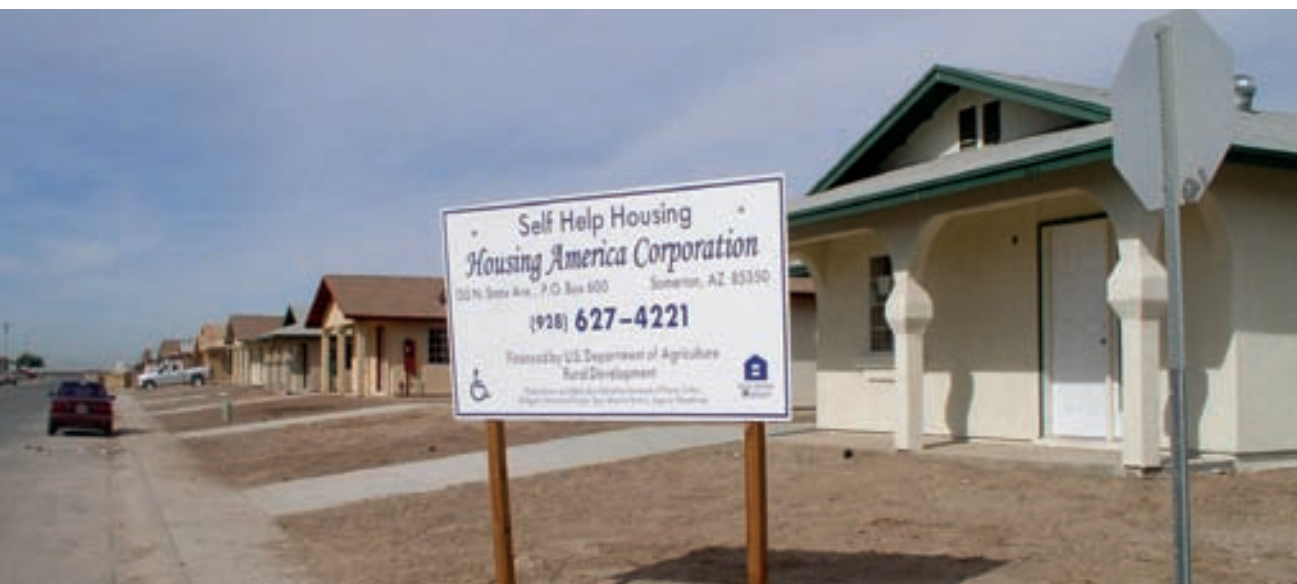
USDA sponsored affordable housing subdivision in Yuma, AZ. The designs are conventional detached suburban houses. Photo: B. Vint
