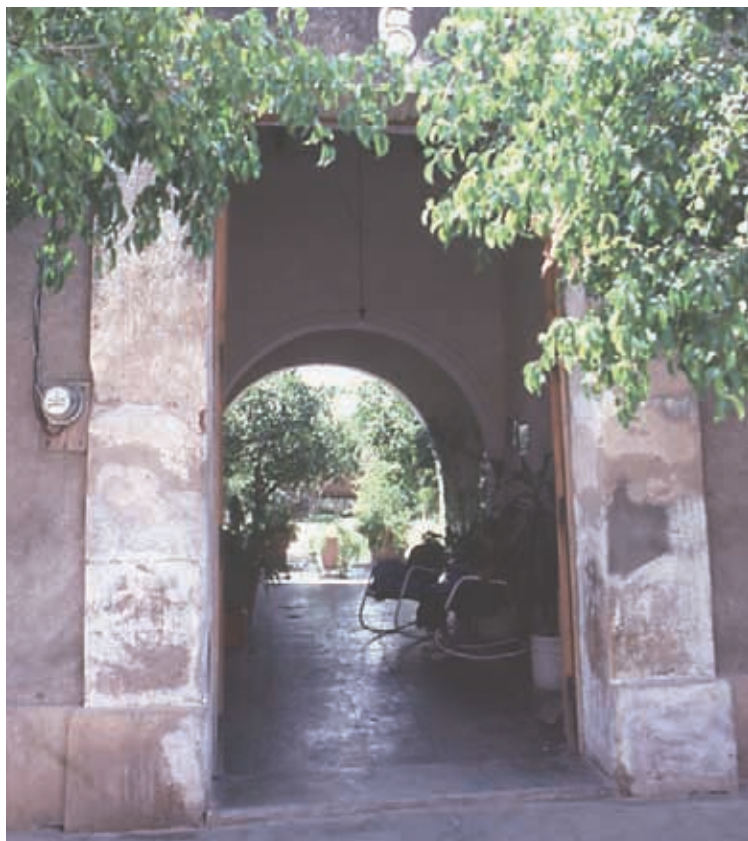
Ures, Son View of zaguán (entry hall) from street. Photo: B. Vint
