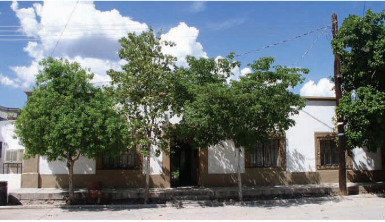
Ures, Sonora: Facade of zaguán house from street. Photo: B. Vint
