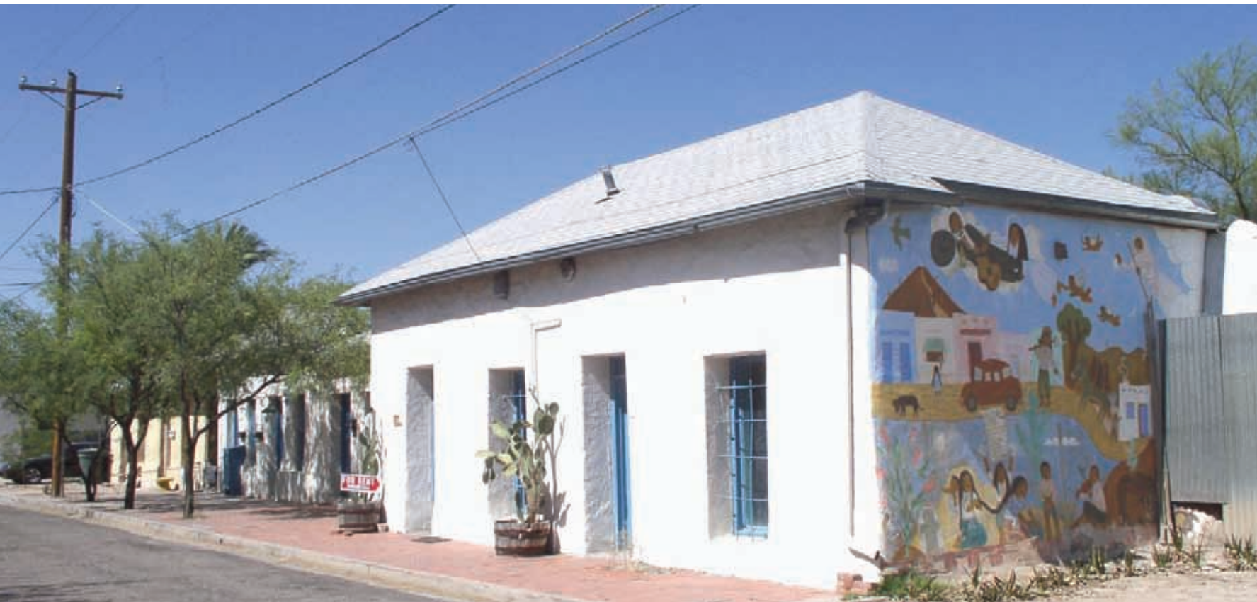
S. Meyer Ave., Barrio Viejo, Tucson: Transformed Sonoran rowhouse. Built ca. 1870 as a simple adobe box, a hipped roof was added in the late 19th Century. Photo: C. Neumann
