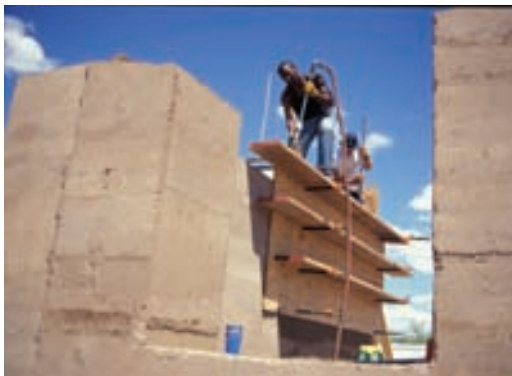
4 Tamping higher portions of wall.
