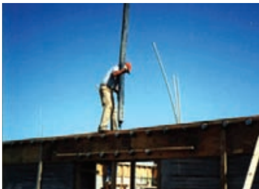
7 Concrete pumped into forms for bond beam.
