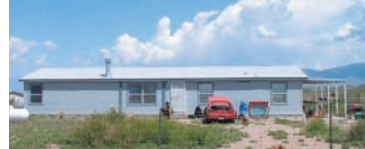
Base case South Elevation Photo: C.Neumann
