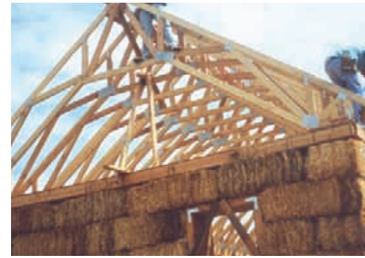
6 Roof trusses mounted to bond beam
