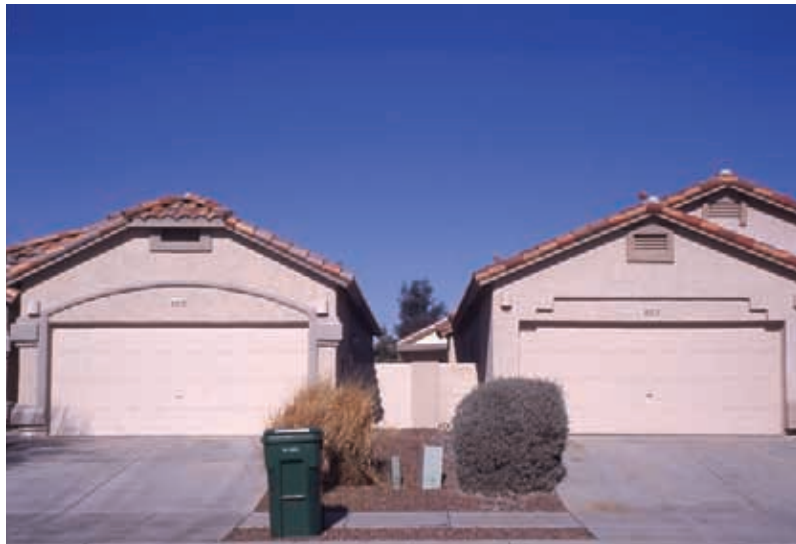
Placement of houses results in side yards which offer neither privacy nor sufficient outdoor space to serve any useful purpose. Photo: B. Vint
