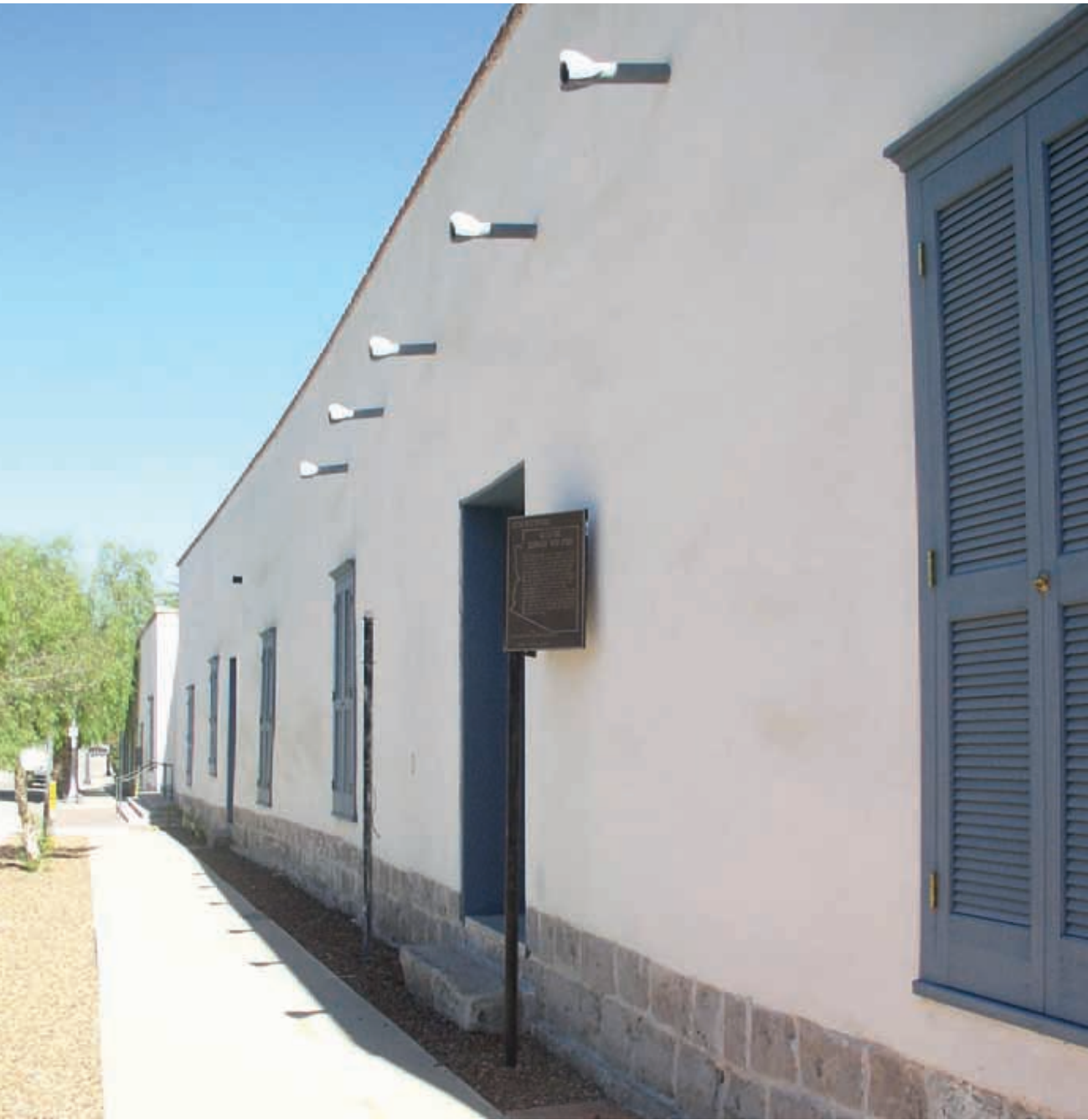
Fortress-like west wall of Fish House provides an excellent thermal barrier against the desert's heat. Photo: C. Neumann
