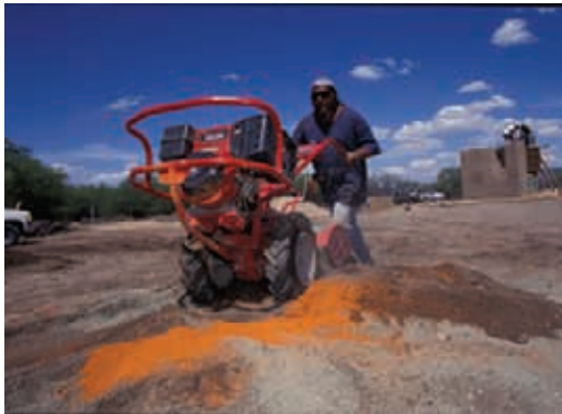
1 Mixing dry soil and cement.
