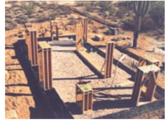
3 Window and door bucks built and set in place.
