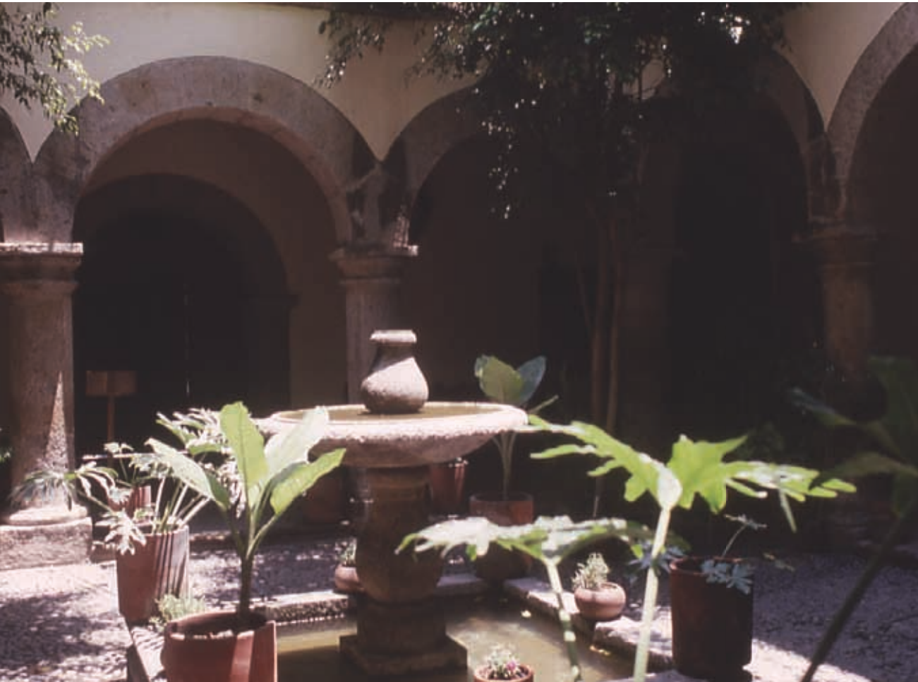
Guadalajara, Jalisco: Courtyard provides evaporative cooling with central fountain and vegetation. Photo: B. Vint
