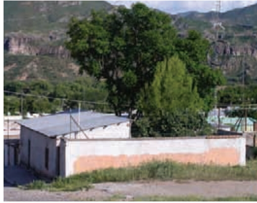
L-shaped house with heavily vegetated courtyard at corner. Photo: B. Vint
