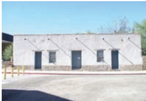
East facade of Cordova House. Photo: C. Neumann
