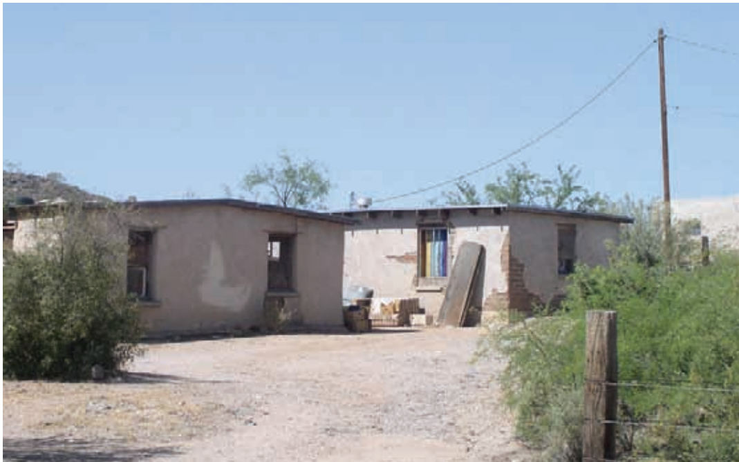
Traditional early 20th century Tobono O'odham extended family housing cluster at San Xavier District. Note adobe walls, minimal wall height and small size of houses. Photo: B. Vint
