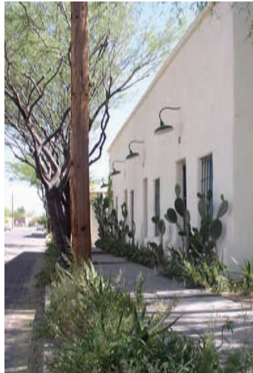
Tucson, AZ: thermal performance of individual units of row house is improved by sharing interior walls and receiving shade from adjacent vegetation. Photo: B. Vint
