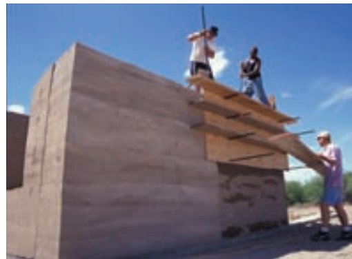
5 Work progressing from building corners.
