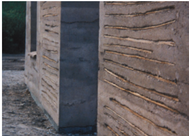
Saguaro ribs integrated into the rammed earth during tamping and anchored by 3” drywall screws and inset on the sides by 12”. The addition of the ribs was debated between students and tribe members since its function is purely ornamental but tribe members deeply wanted to maintain ties to traditional sandwich wall construction. Photo courtesy of M. Hardin
