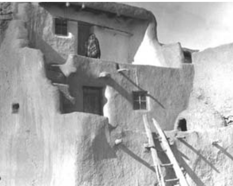
South facing roof terraces at Acoma Pueblo ca. 1935. Photo: F. Hannab by permission of Arizona State Museum
