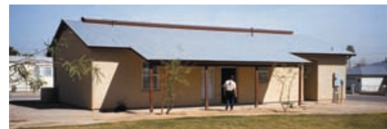
Guadalupe, AZ: 1,100 sf three bedroom, load bearing straw bale home financed by HUD for a low-income family in 1997. 160 volunteers raised the bale walls and framed and sheathed the roof in a single day. The interior and exterior stucco was done later. This project was a joint effort of HUD, The Development Center for Appropriate Technology (DCAT) and Out-On-Bale (un)Ltd. Photos courtesy of M. Myhrman & J. Knox
