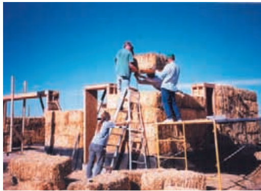
4 Volunteers erect bale walls on workday.
