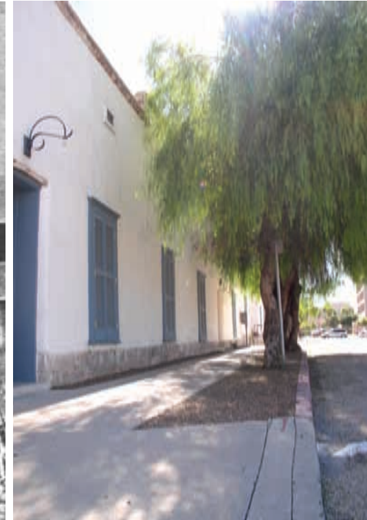
Shutters and Pepper trees provide shade at west facing wall. Photo: C.Neumann
