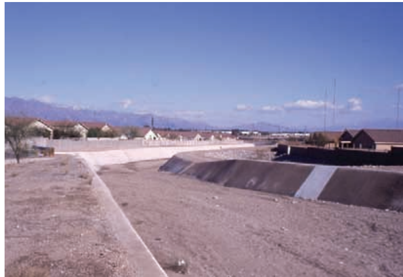
Civil engineering to accommodate rain runoff from streets and roofs leads to concrete-lined drainages as public spaces. These developments are technically adequate, but raise environmental and aesthetic issues. Photo: B. Vint
