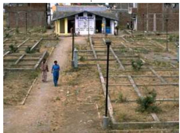
Fig -6: plinth constructed for EWS
