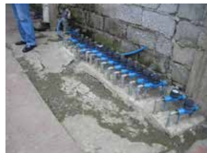
Water connections: Metro Manila, Philippines Photo: B. Banerjee
