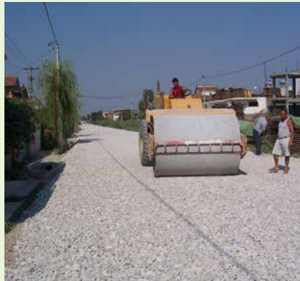
Residents organize themselves with support from the NGO CoPlan in the execution of their street plan using gravel pavement and compacting. A successful practice in the informal areas of Tirana, Albania . © Coplan.
