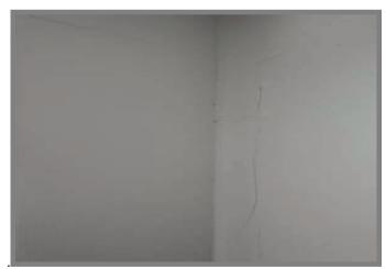
Figure 2. Hairlines cracks on internal walls
