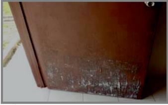
Figure 6. Peeling paint on door
