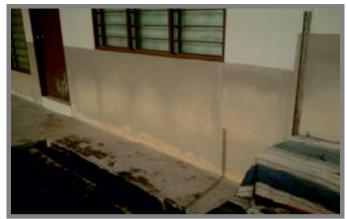
Figure 5. Discoloration on wall area
