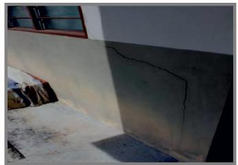
Figure 3. Vertical cracks on an external wall
