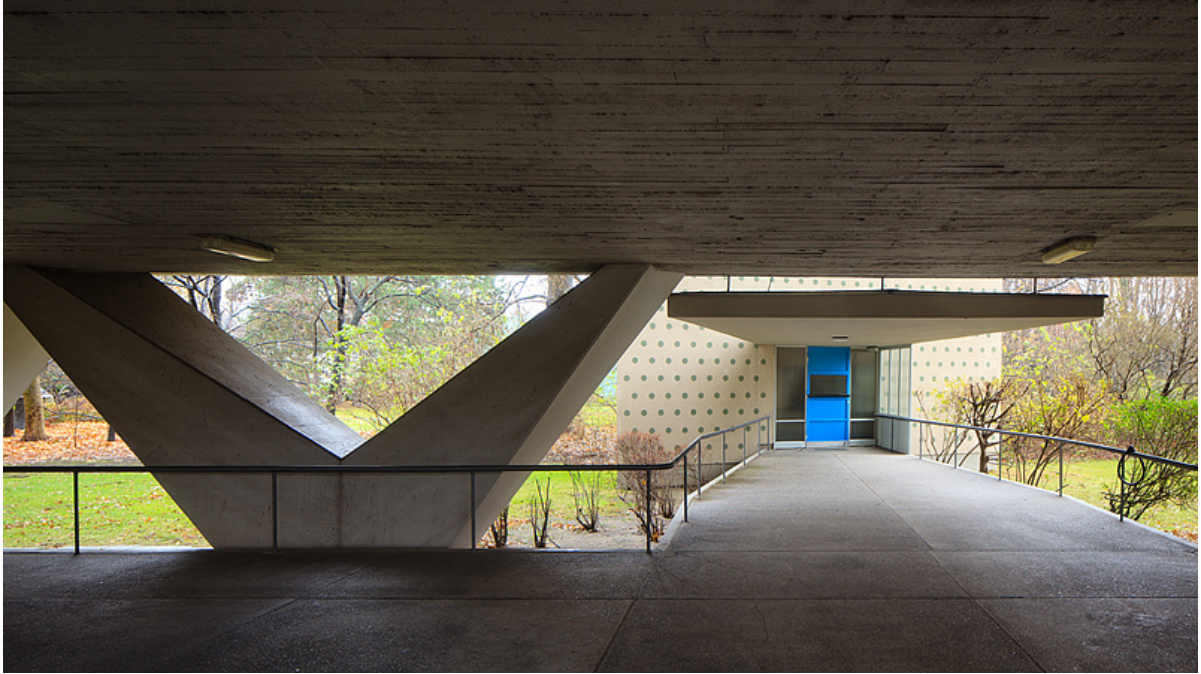
Figure 38 Interbau House open ground floor looking to elevator tower
