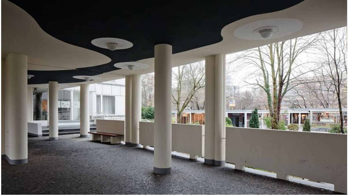
Figure 44 Klopstockstrasse ground floor common area
