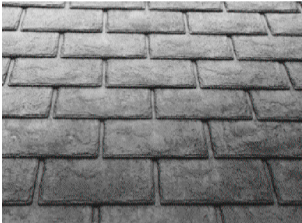
Figure 23: Fiber-resin composition roofing tiles cast from 100-year-old slates for an authentic look.
