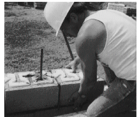
Figure 10: Concrete blocks with foam inserts.
