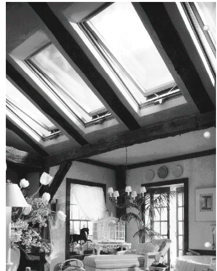
Figure 21: Operable skylights provide daylighting and natural ventilation.
