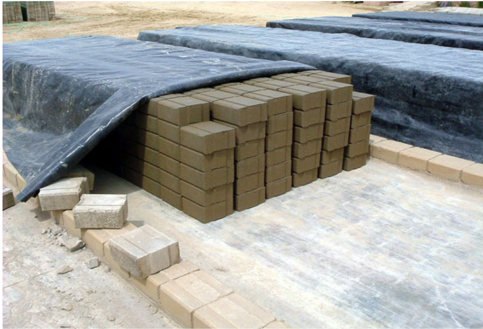
Figure 2: Stacking of Solid Interlocking blocks. Source: Field survey (2007)
