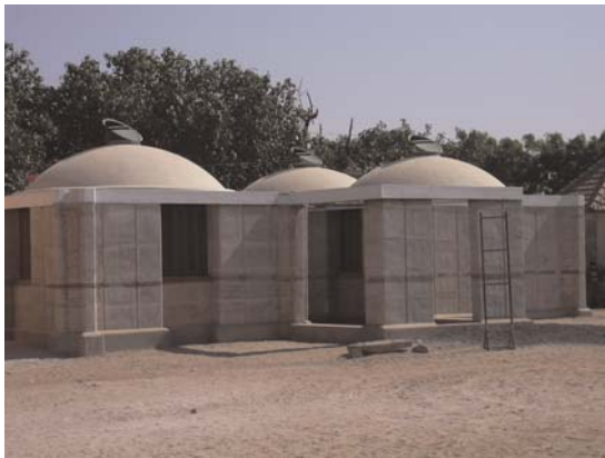
Figure 3. Load-bearing stabilized rammed earth building.
