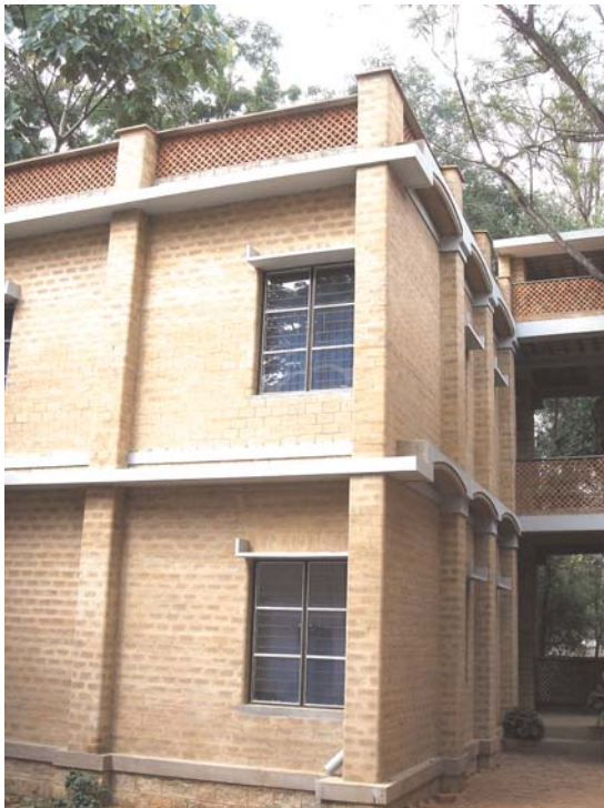
Figure 1. Load-bearing SMB masonry building.
