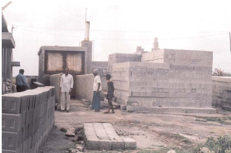
Figure 2. Small-scale compacted fly ash block manufacturing unit.
