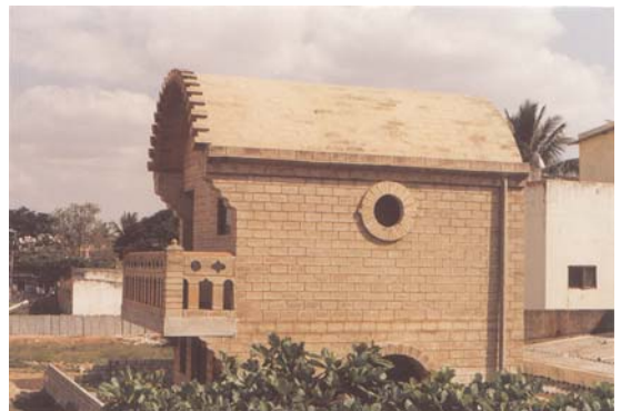
Figure 6. Unreinforced SMB masonry vault roof.
