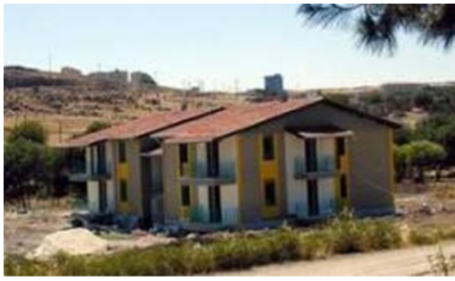
Fig. 3. Alker Building, four apartments on 2 stories at Urfa, Turkey [38].
