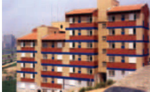
Image 12: Some of the Cingapura blocks located on the area with land slide risk
