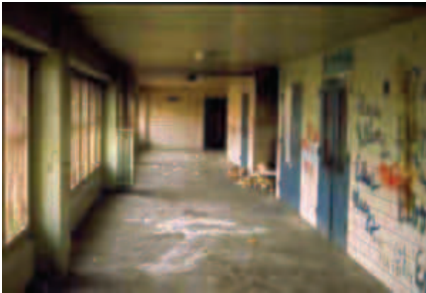
Image 1: Actual 3rd floor communal corridor of the Pruitt Igoe Social Housing buildings 10 years after the construction in 1954, ghettoization.
