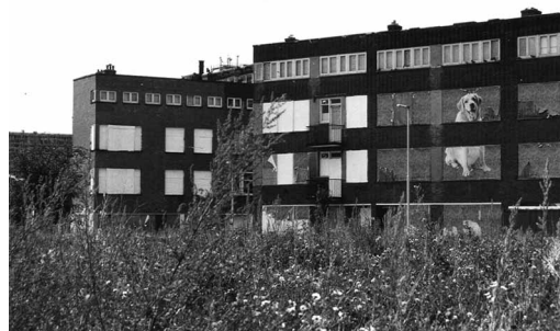
Figure 11. More blocks will be renovated in the next few years.
