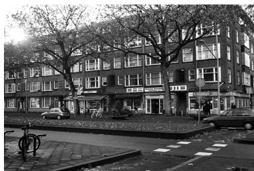
Figure 7. The Dordtselaan forms the border between the city districts of Charlois and Feijenoord. In the past, it received little attention because both districts did not consider it their 'prime territory'. With the renewal of the Millinxbuurt, problems such as drug dealing and milking properties cross the Dordtselaan and pop up again in Bloemhof, the neighbourhood on the other side of the street.
