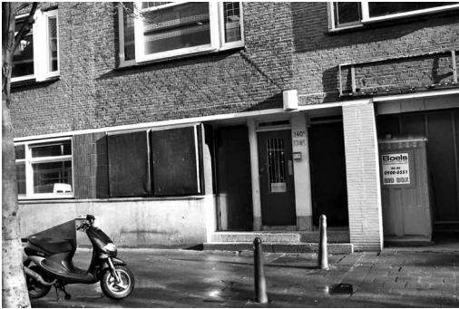
Figure 12. The city district and the local police check all buildings and, in case undocumented immigrants are accommodated or the building is used for drug dealing or drug using, it will be closed with a steel door and steel windows to prevent people from entering.
