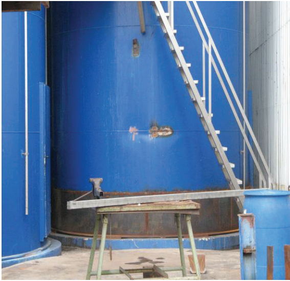
Figure 11(a): Repaired Steel Tank
