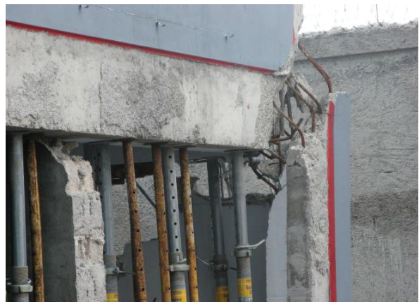
Figure 3: Beam-Column Joint Failure
