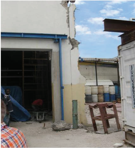
Figure 4: Interrupted Shear Wall
