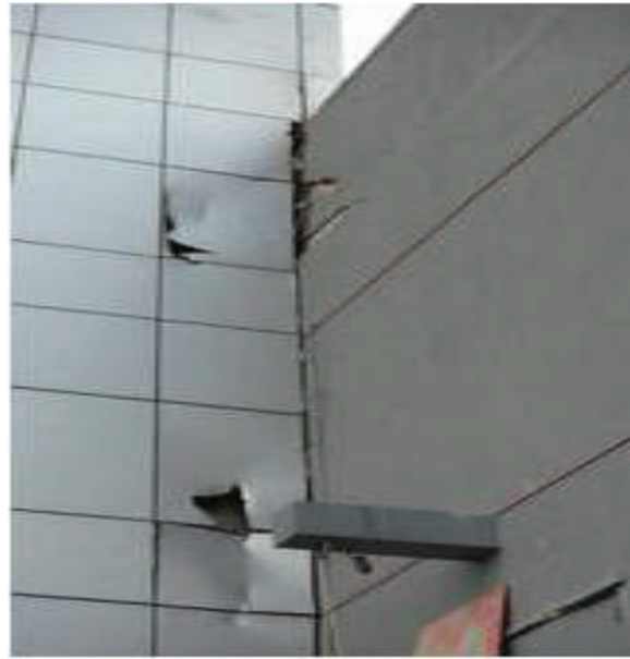
Figure 5: Pounding Failure
