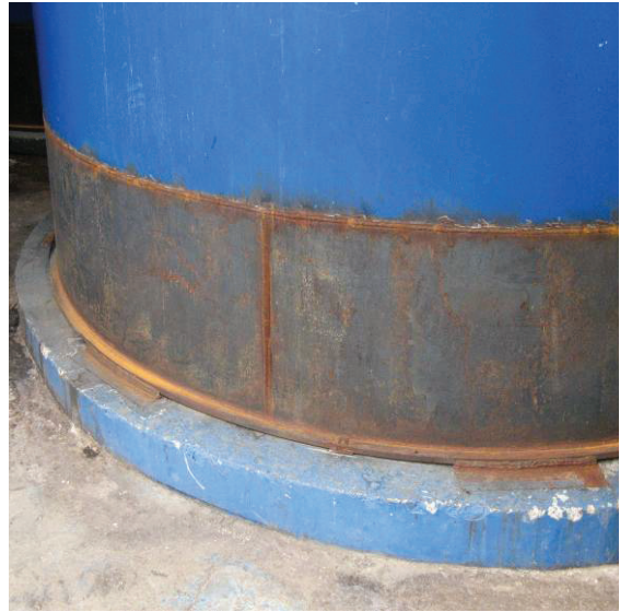
Figure 11(b): Repair at Base
