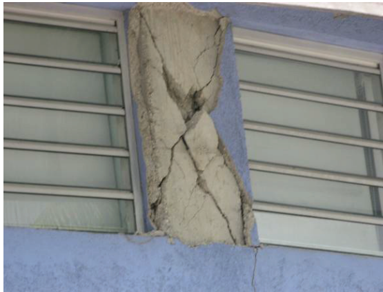
Figure 1: Failure of Captive Column, Exterior and Interior
