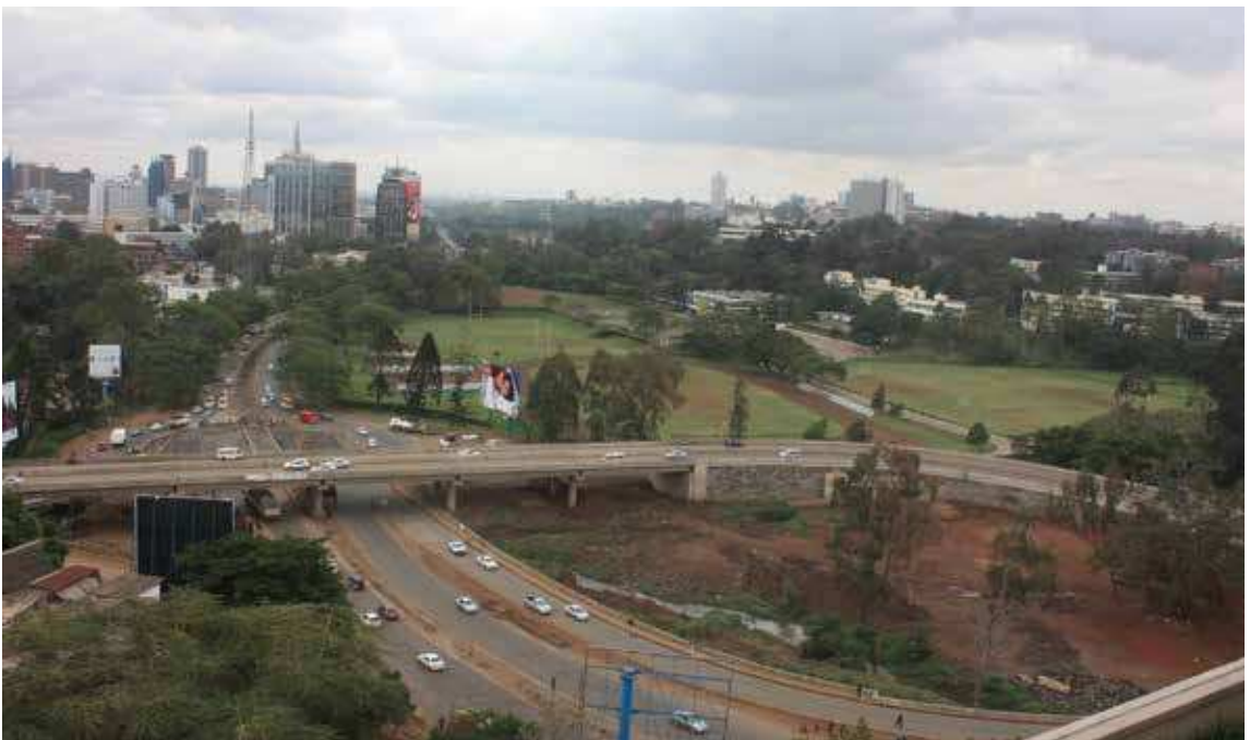
Construction of infrastructure in Nairobi, Kenya © Kenya Vision 2030
