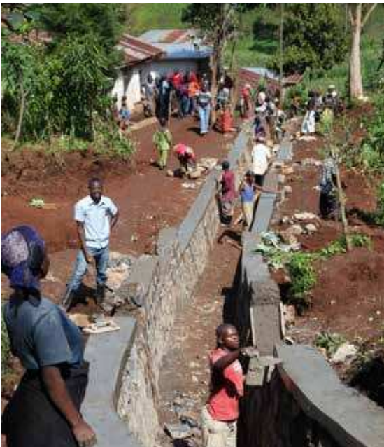
Construction of water tunnel in Rusizi, Rwanda © UN-Habitat/Julius Mwelu
