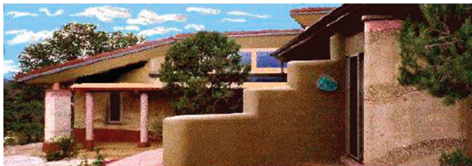
Figure 2: The first Cast House, Prescott, Arizona, USA, 1996. Source: Cast Earth Website.
