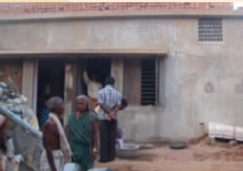
Picture 2 : A house under construction in Bhubaneswar.
